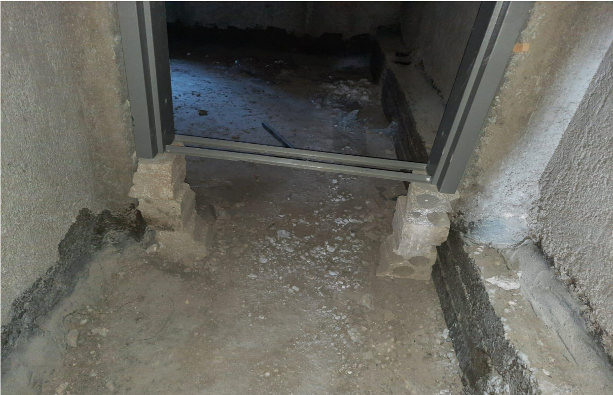
Door frame supported by blocks
