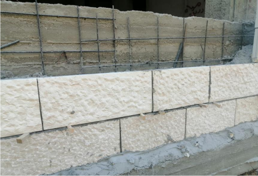
An example of acceptable stone building
