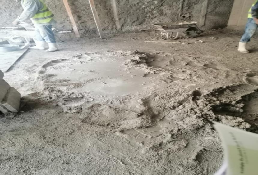
Preparing the mortar mix without using special container
