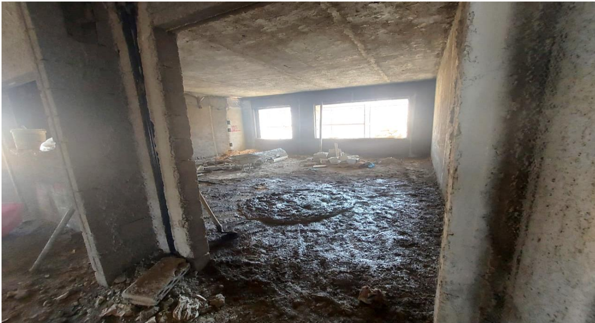
Mixing mortar without using a container
