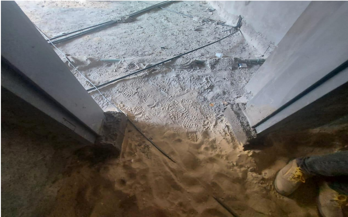
Casting concrete under the door frames
