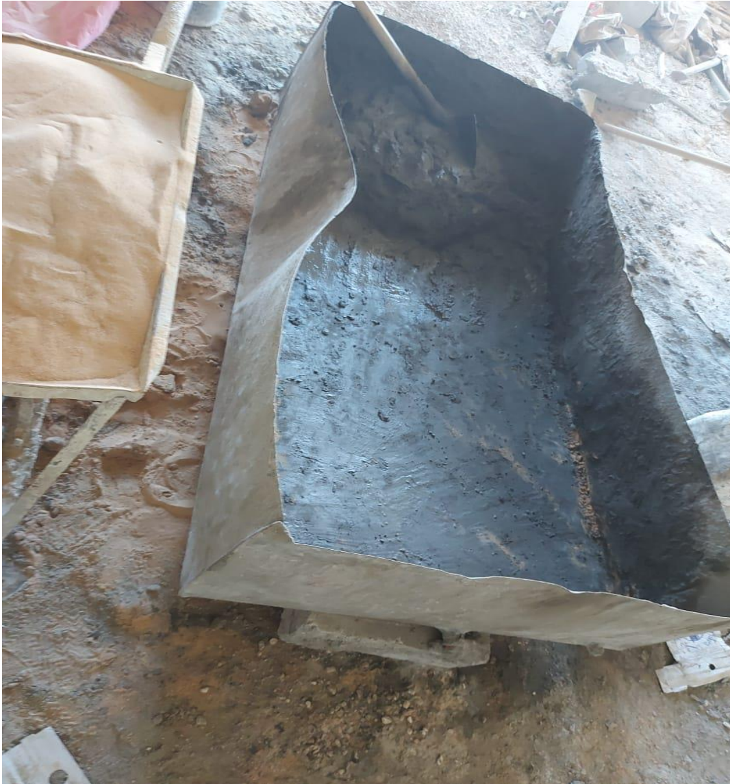
Mixing mortar by using a container
