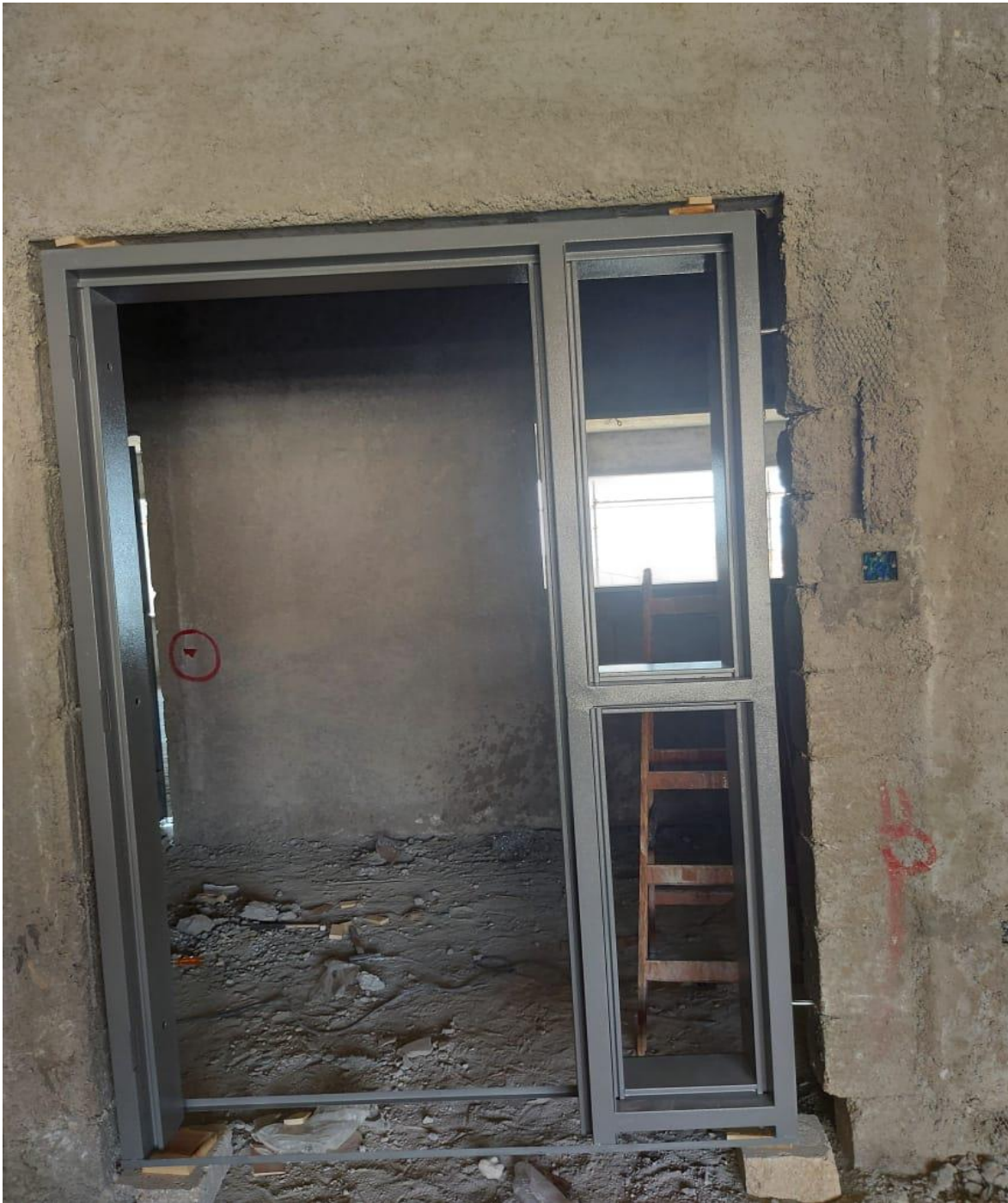
Door frame supported with block
