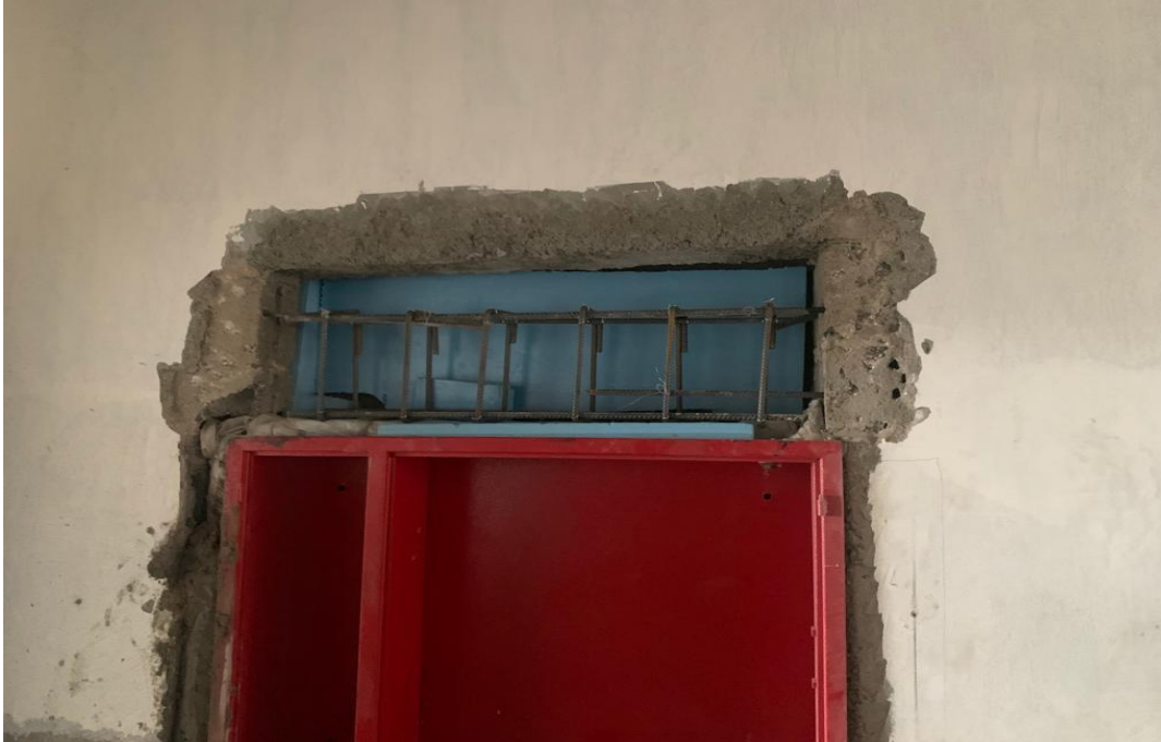
Steel reinforcement for lintel over the fire hose cabinet
