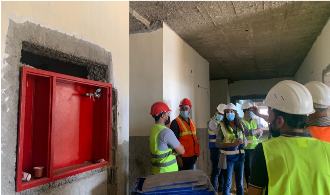
Space over the fire hose cabinet needs to be casted
