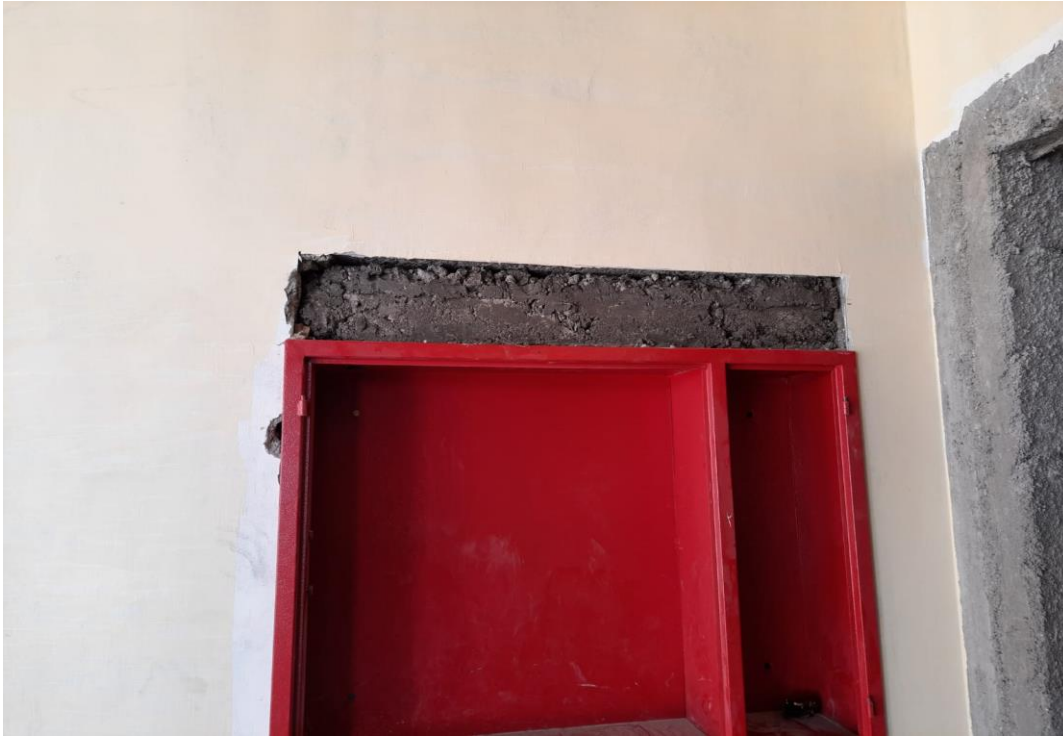
Casting concrete for the lintel over the fire hose cabinet
