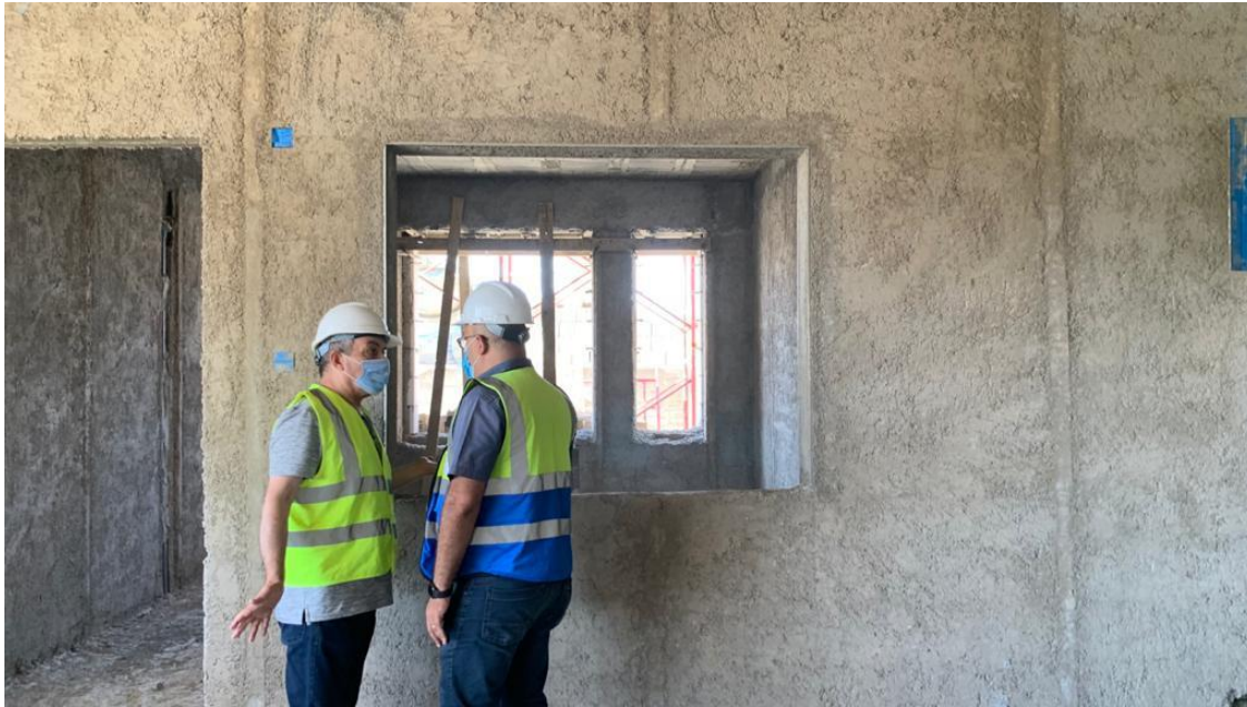
Plastering beads are used for windows' edges
