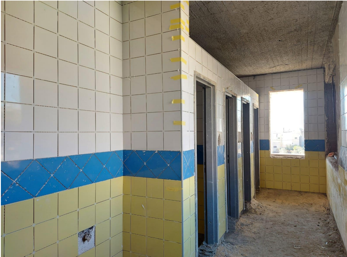
Tiling work at the wet area (figures: 22, 23, 24 & 25)
