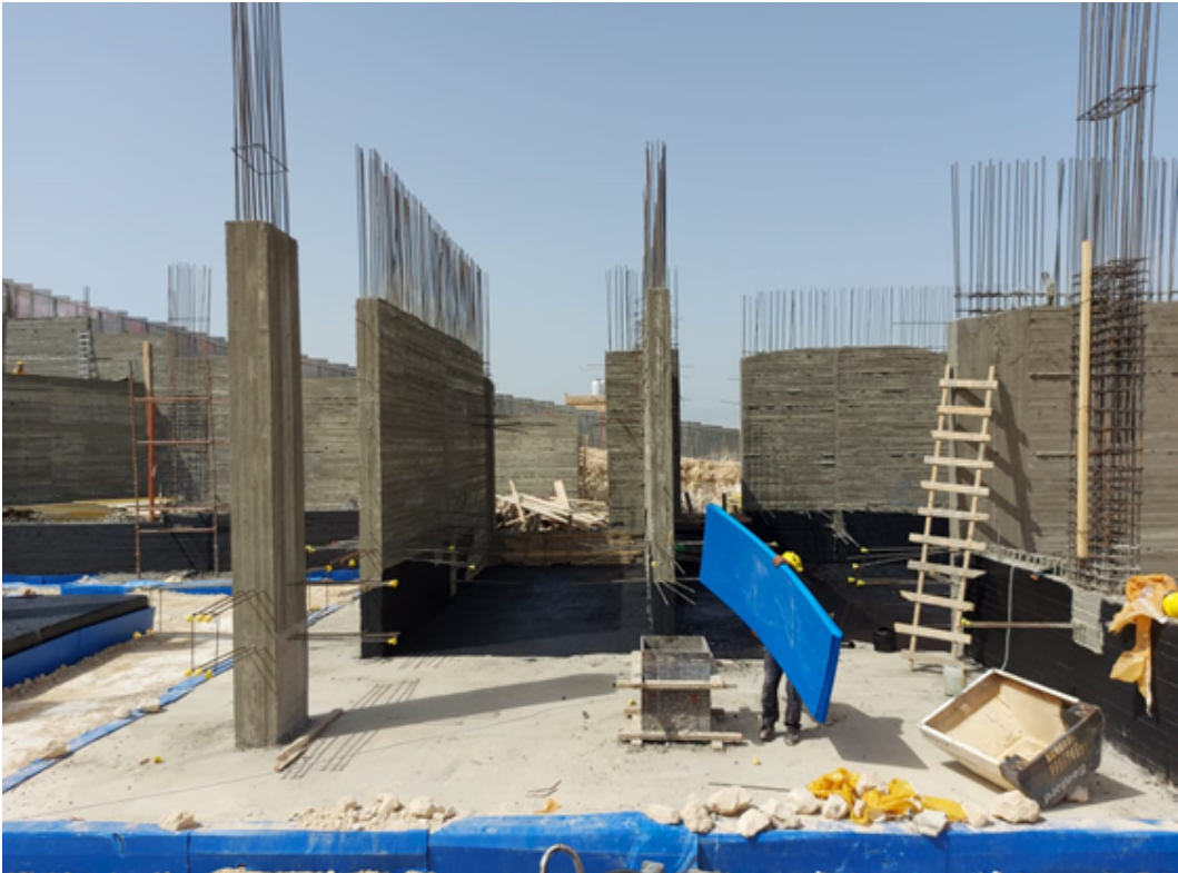
Dismantling of columns formwork- (22/03/2021)
