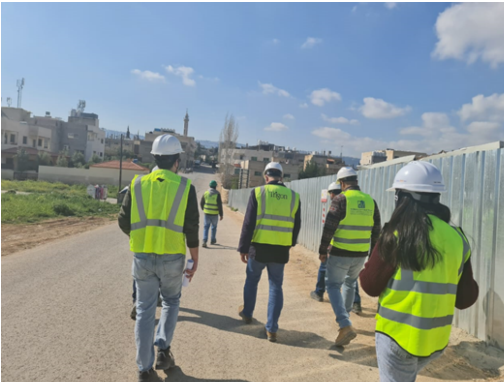
Checking the encroachment of the existing street toward the school land
