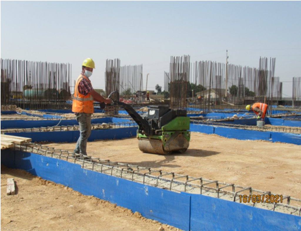
Back-filling compaction- (16/03/2021)
