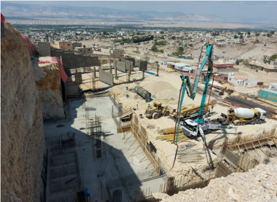
General view of the Project- (28/03/2021)
