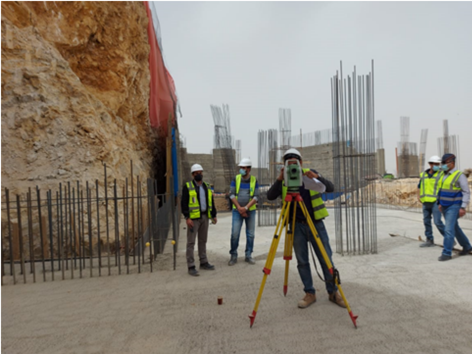
Surveying works on site
