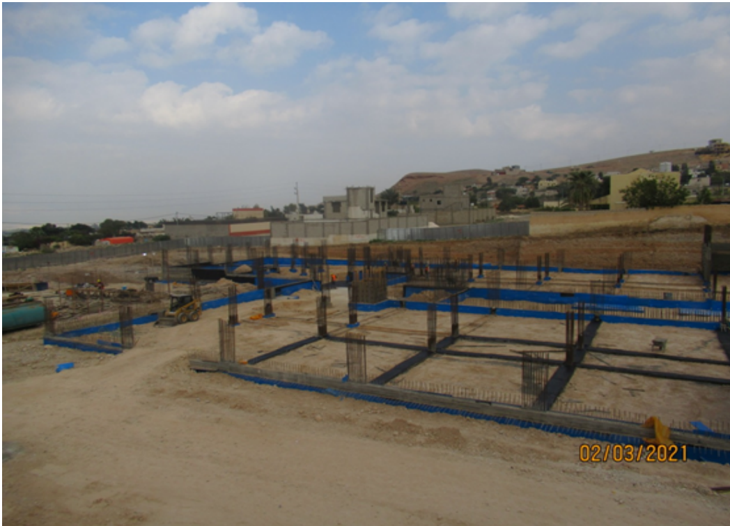
General view of the work below slab on grade- (02/03/2021)
