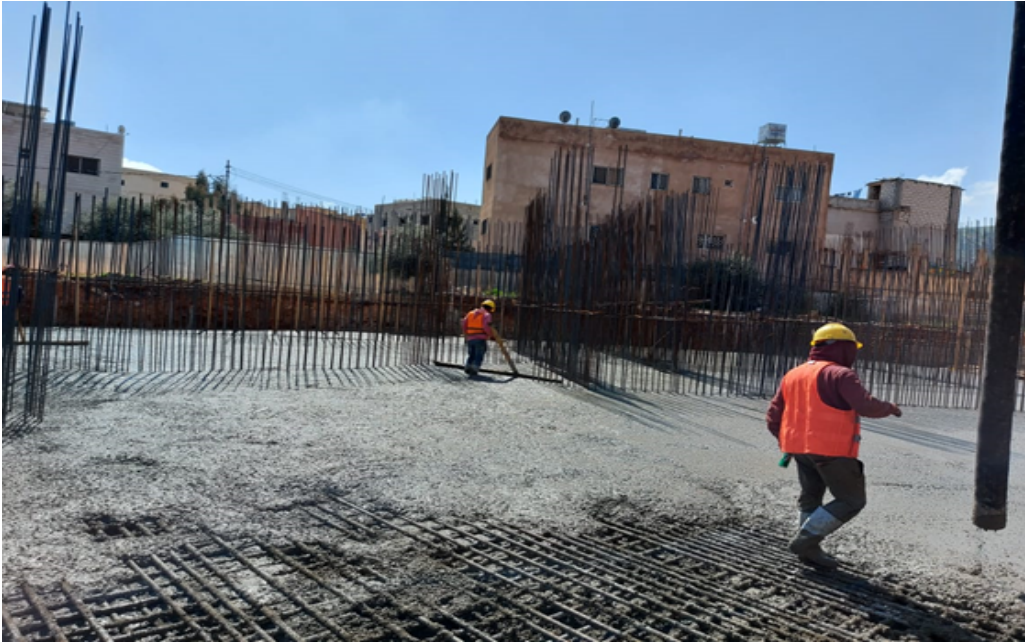
Concrete casting for raft foundation 3&4-(02/03/2021)
