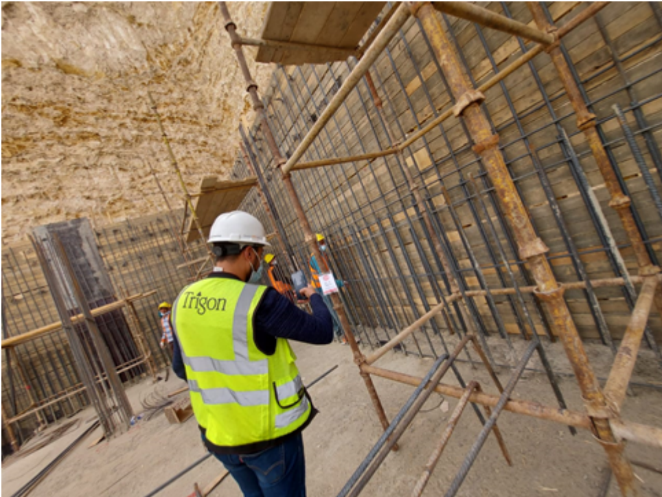
Retaining wall for the main building
