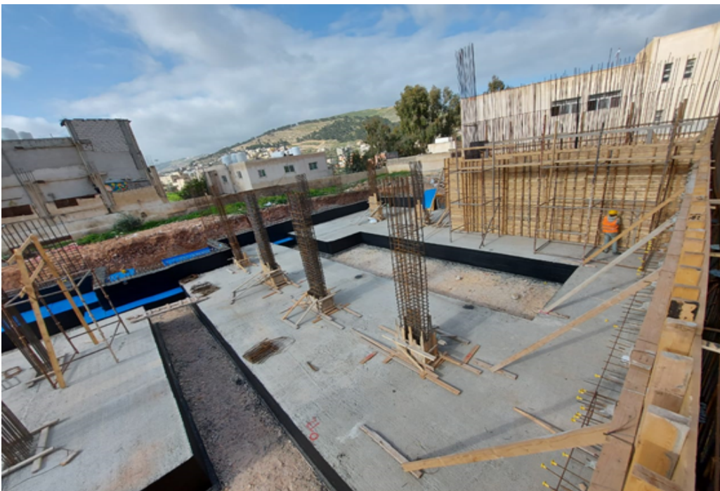
Erecting formwork for columns neck and basement walls- (08/03/2021)
