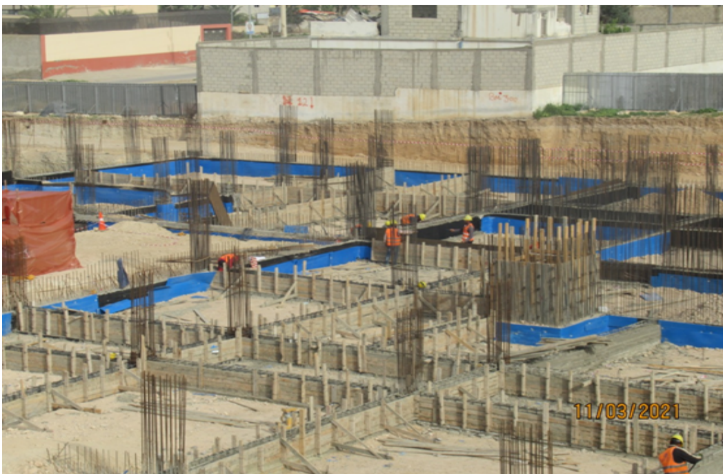
Preparing of formworks for ground floor- (11/03/2021)
