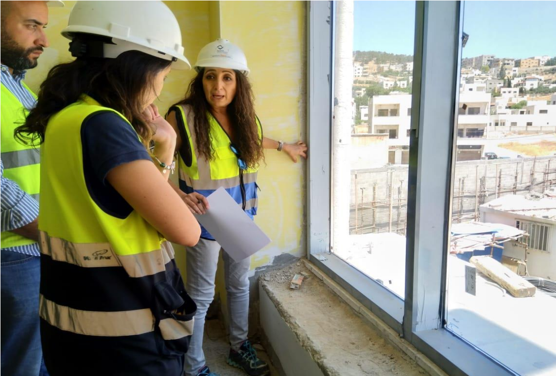
Wrong installation of curtain wall
