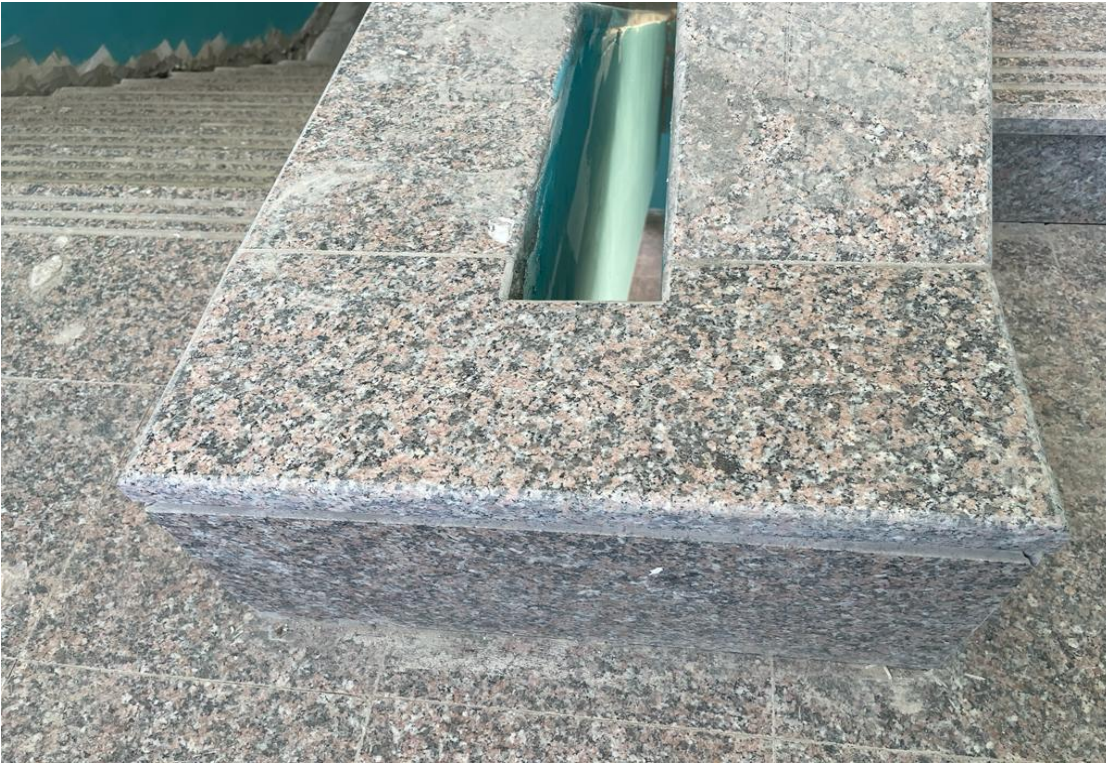
Replacement of small pieces
