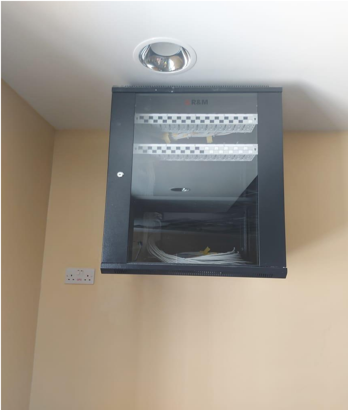
Repair of patch panel cabinet
