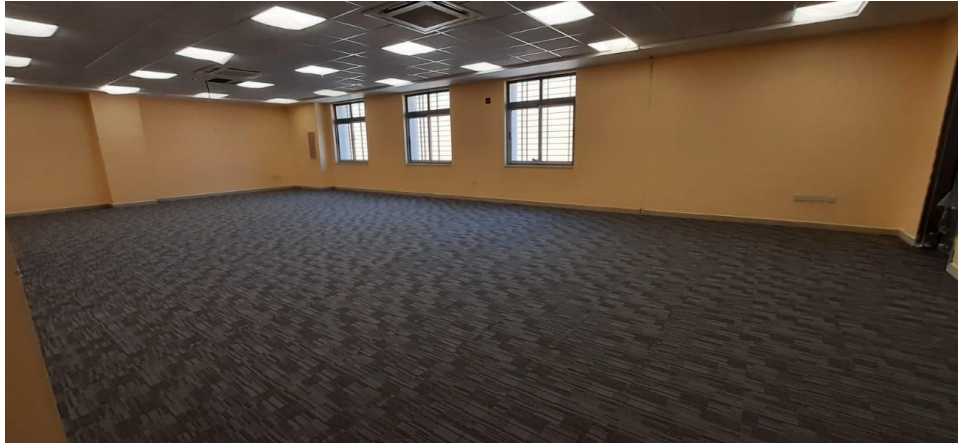
Installing the carpet at the library
