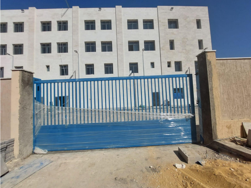
Installing the main steel gate for the parking area
