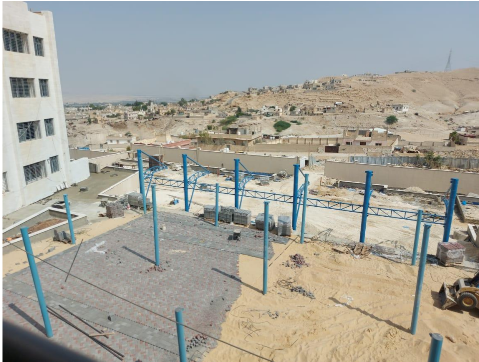
General view of the external works
