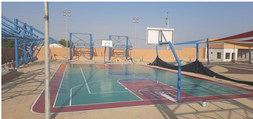
Painting work for the playground
