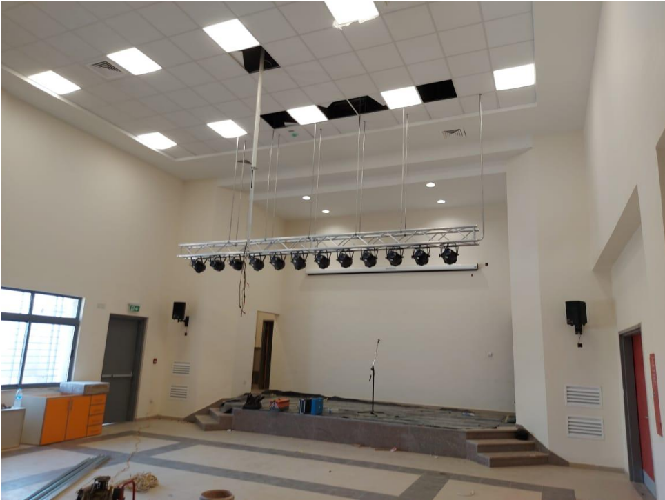
Finish works at the multi-purpose
