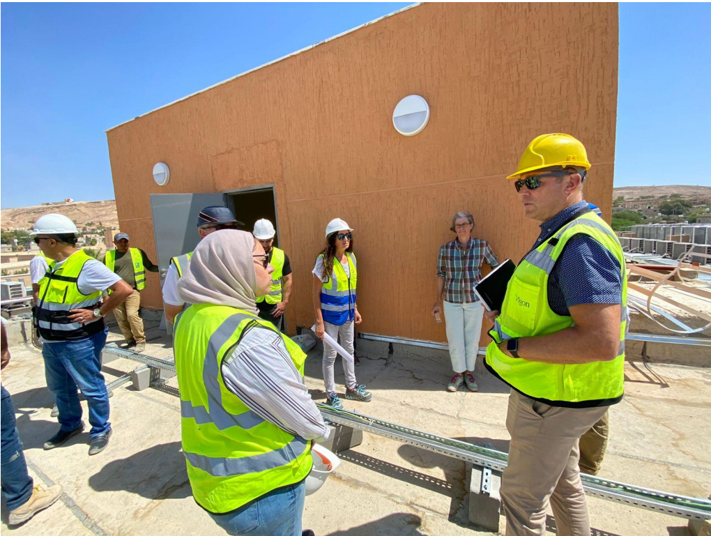
Works at the roof
