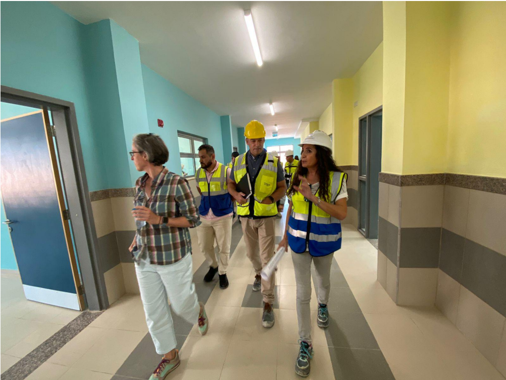
Works at the corridors
