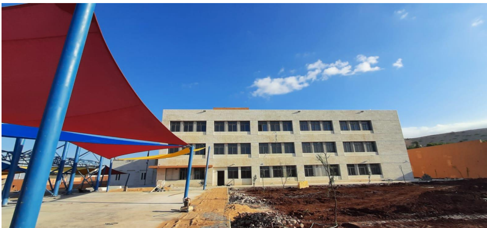
Filling planters with soil and tensile shadings at the external yards
