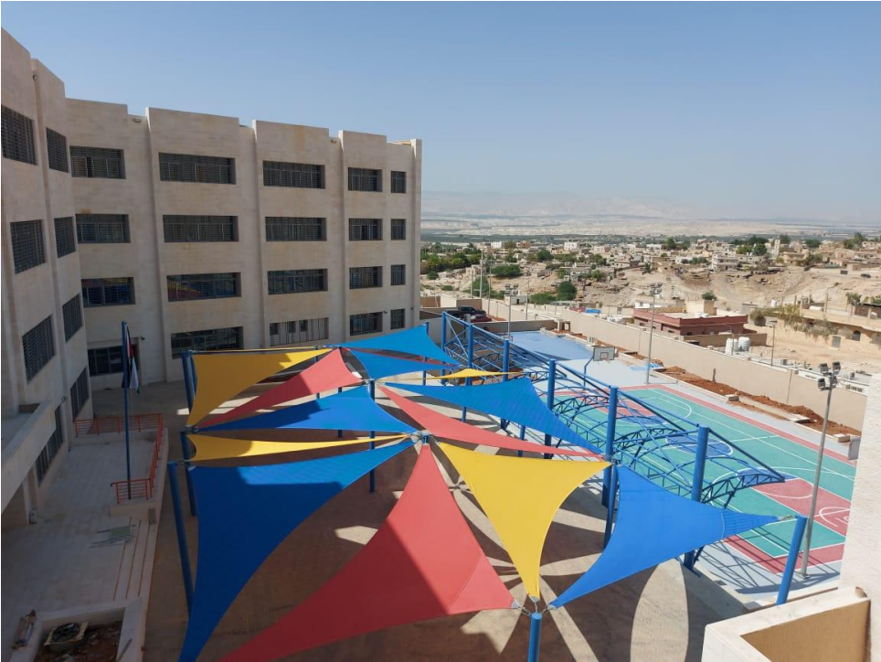
General view of the external works
