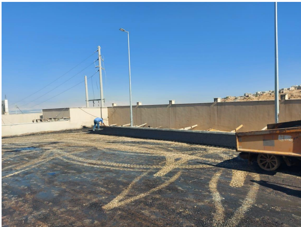
Applying the MC coat for asphalt at the parking area
