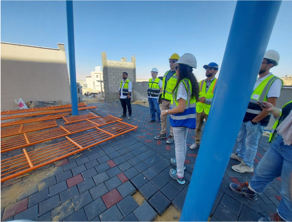
Inspecting the external works
