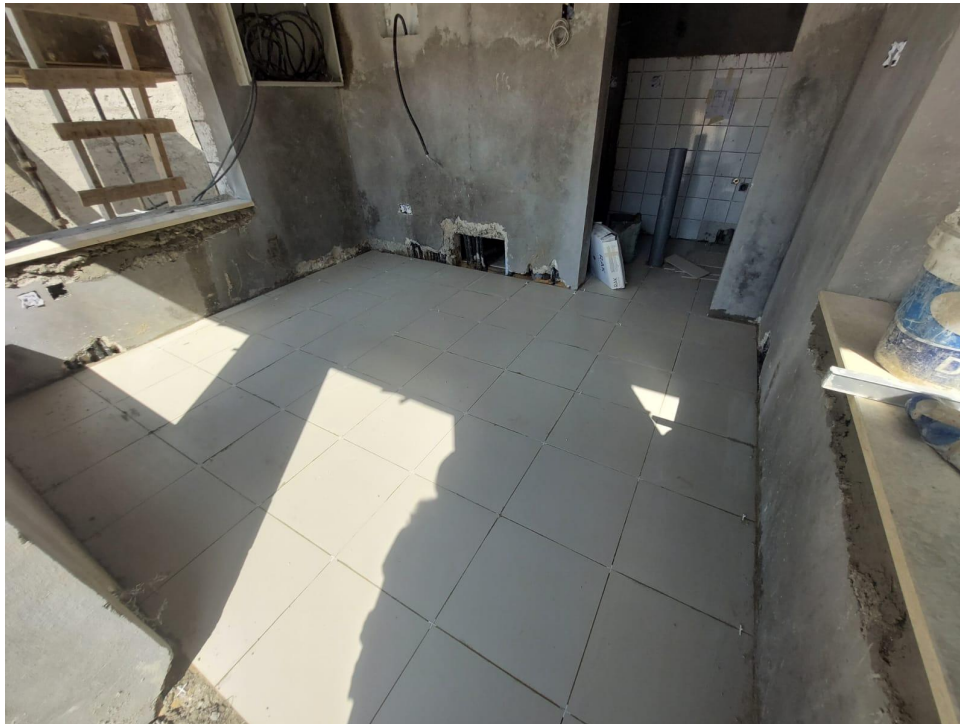
Tiling, plastering and electrical works at the guard house
