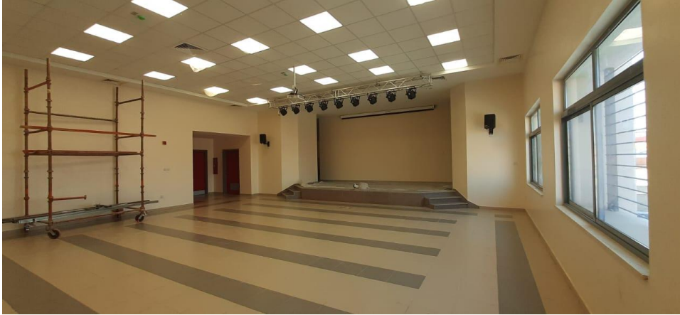
Works at the multi-purpose hall
