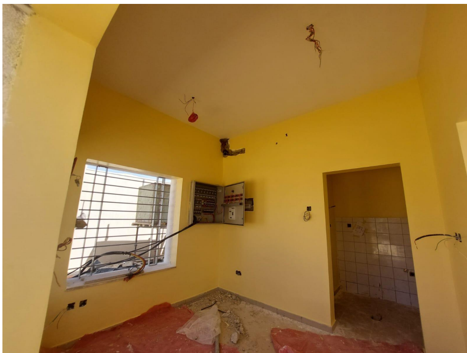
Finishing tiling, painting, and electrical works at the guard house
