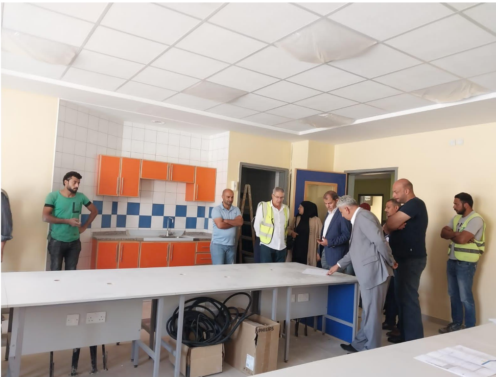
Inspecting delivered and installed furniture
