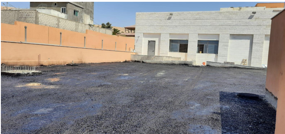
Applying the MC coat for asphalt at the parking area
