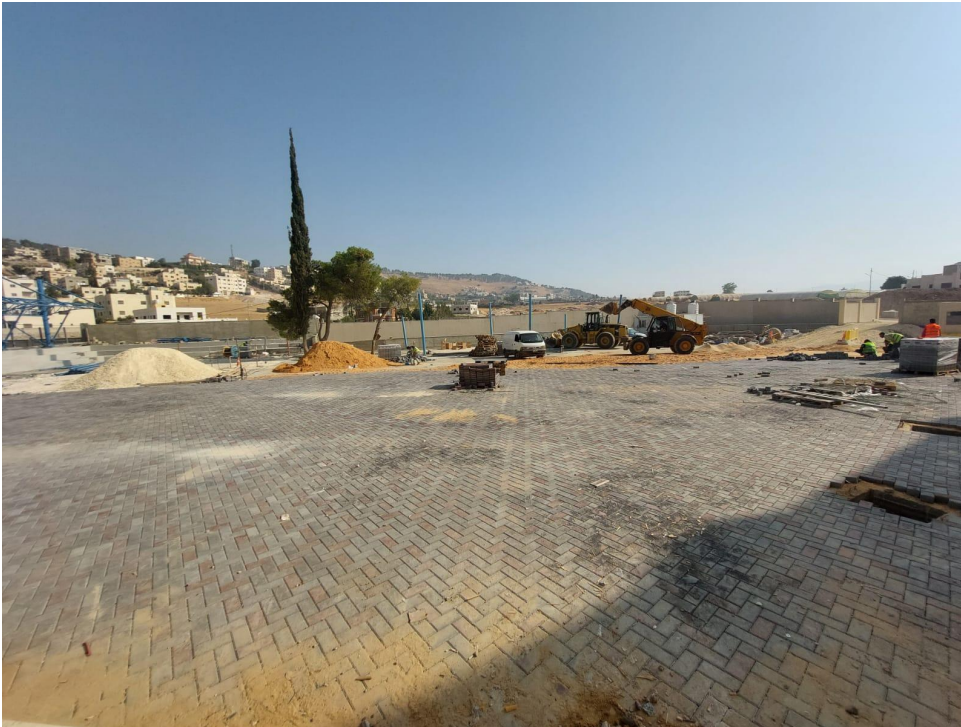
Interlock tiling for the external yards
