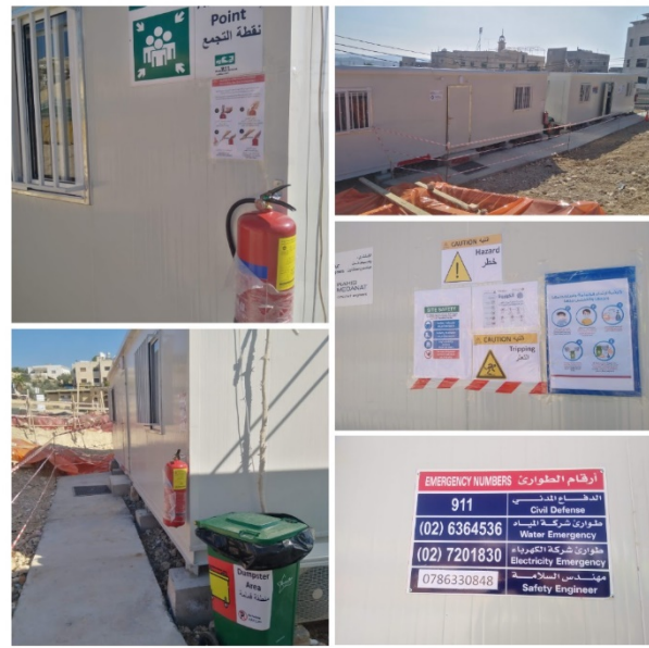
Figure #5: Fire extg., emergency contact numbers, safety signs and other safety devices available; Waste containers provided; Assembly point identified; and Publications on prevention and control of the spread of the COVID-19 were distributed in all project facilities. Photo credit: Odai Tawalbeh, 11/18/2020
