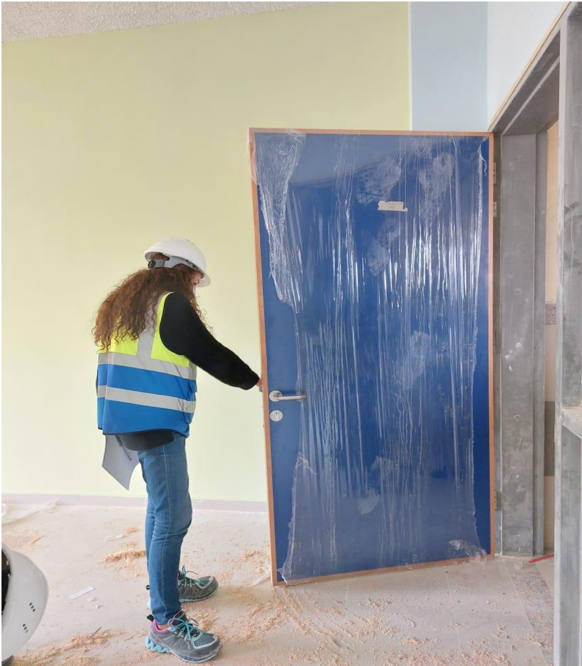
Defected beech wood frames
