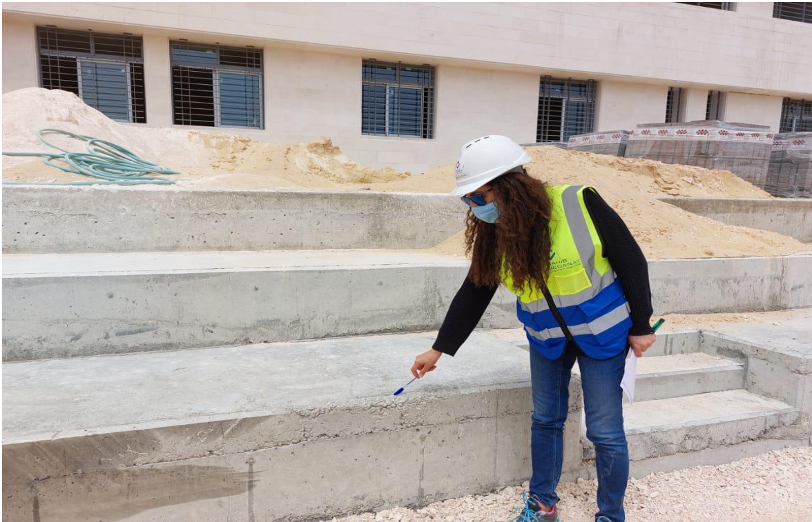
Defects in concrete
