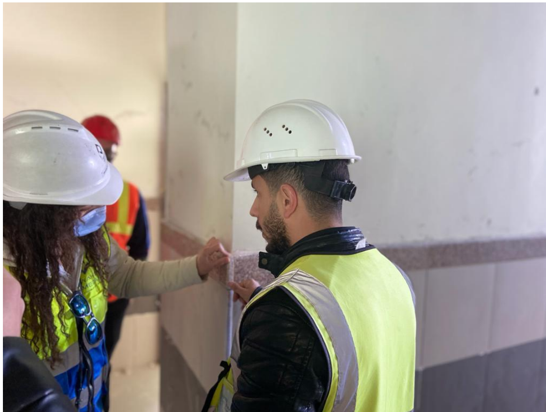
Discussing the execution of granite coping at the corners.
