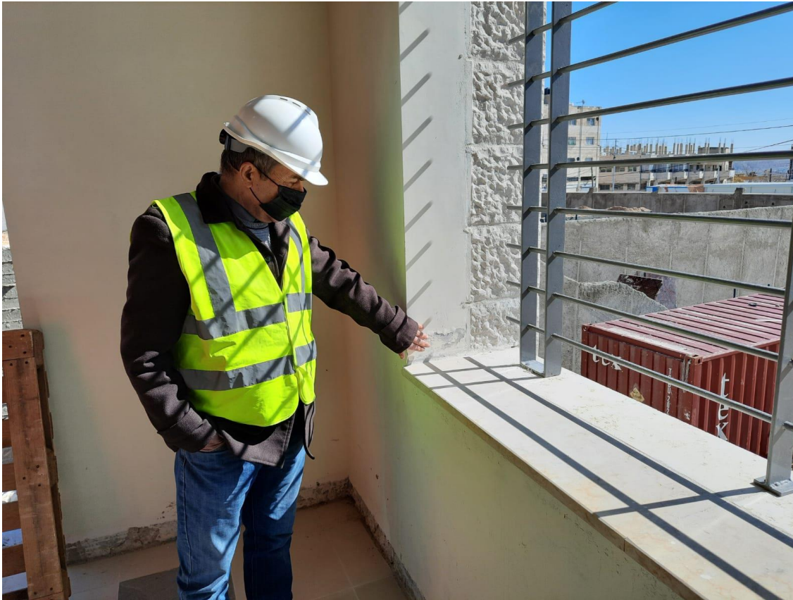
Inspecting the finishing work for window jambs.
