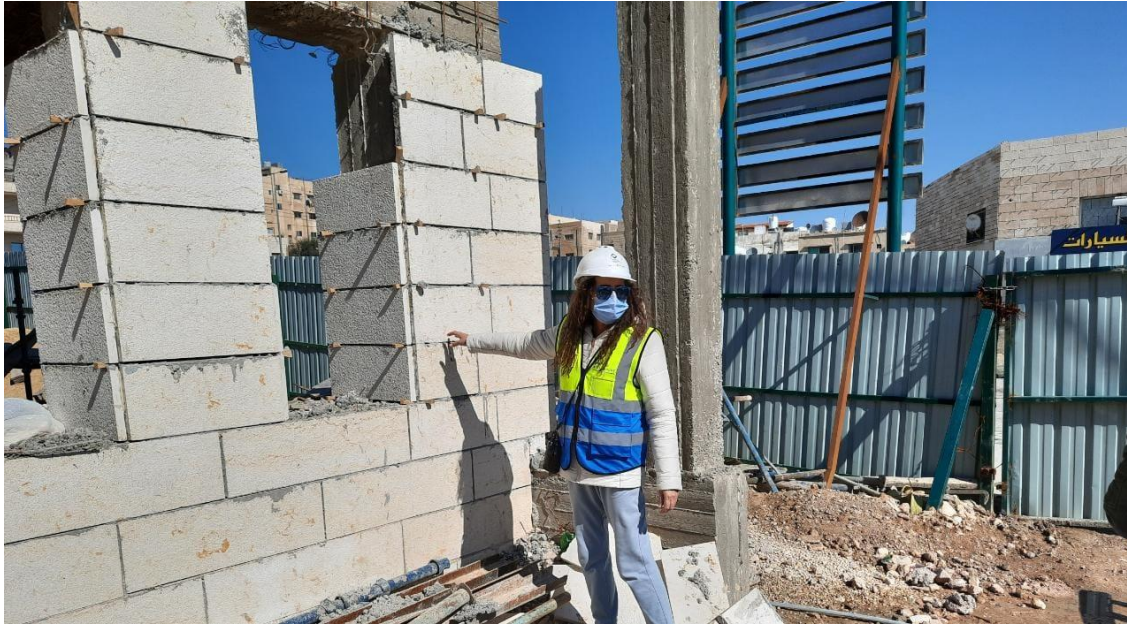
Inspecting the built stones for the guard room.
