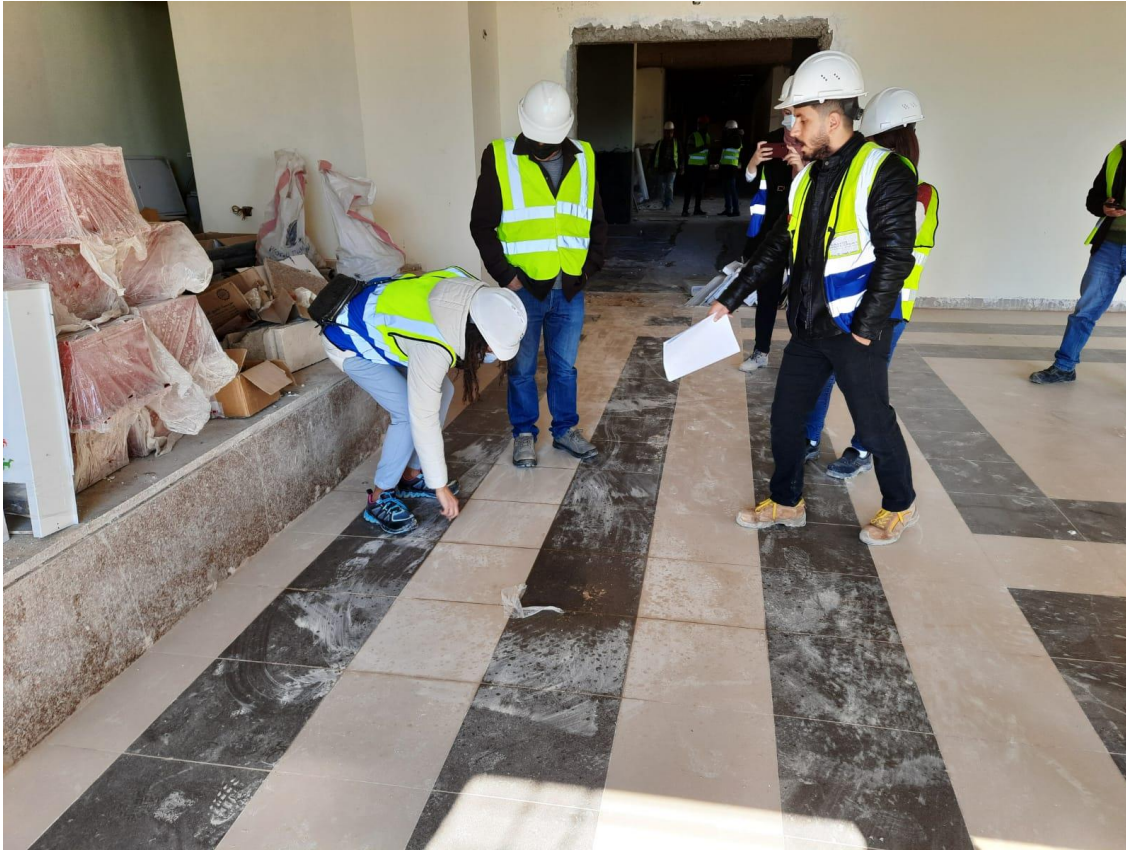
Inspecting the porcelain floor tiles at the multi-purpose hall.
