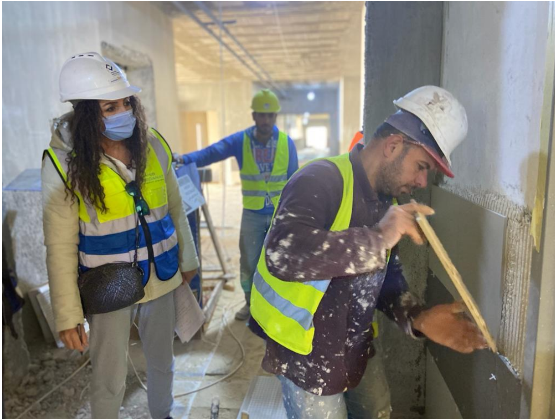
Inspecting the tiling at the corridor's walls.
