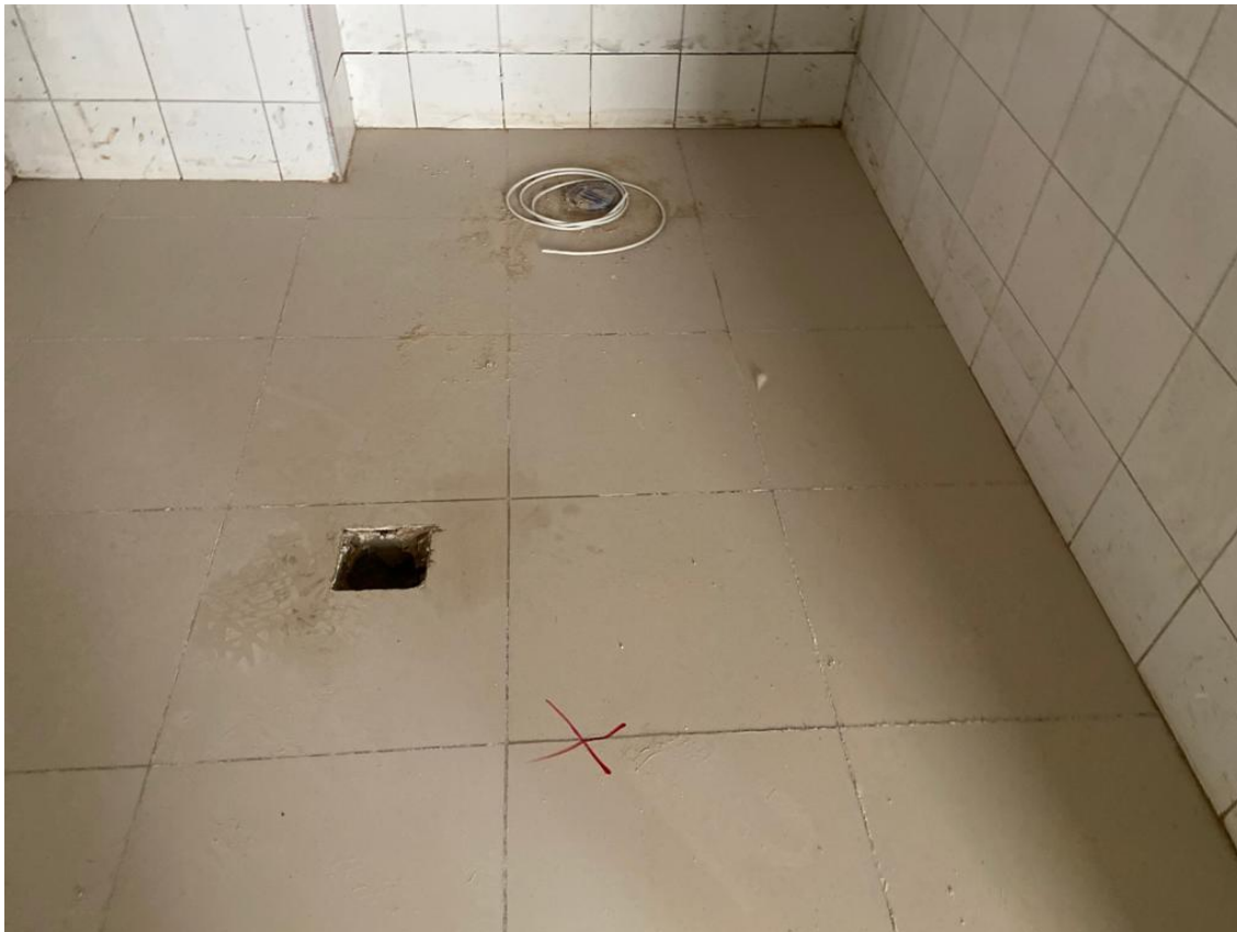
Inspecting the floor drain and clean out location
