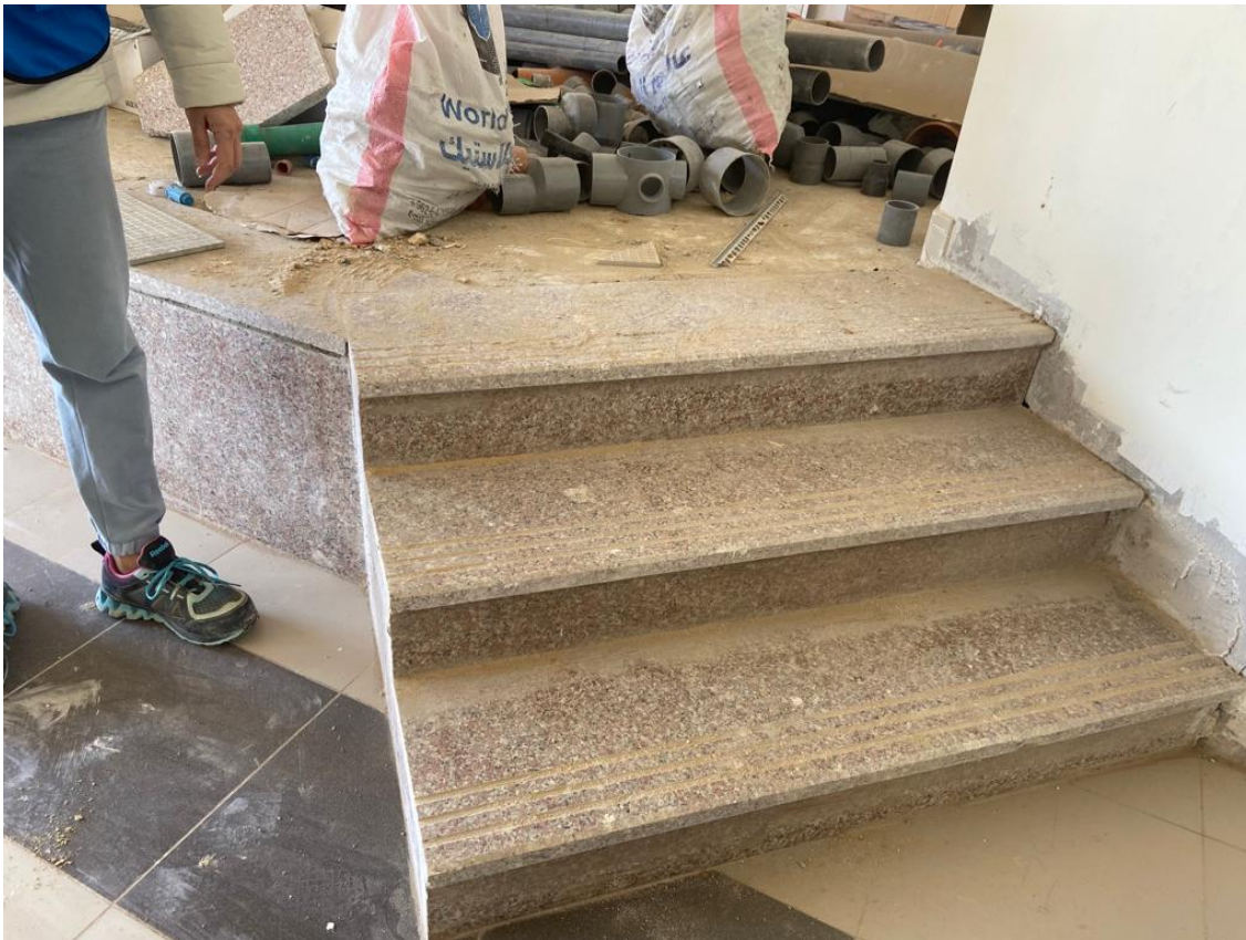
Inspecting the executed stairs at the multi-purpose halls.
