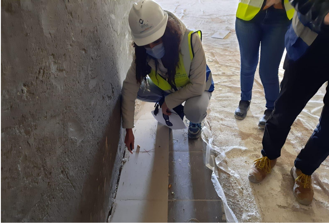
Defected floor tiles at the corridors
