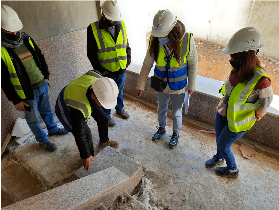
Inspecting the executed granite for staircase parapets
