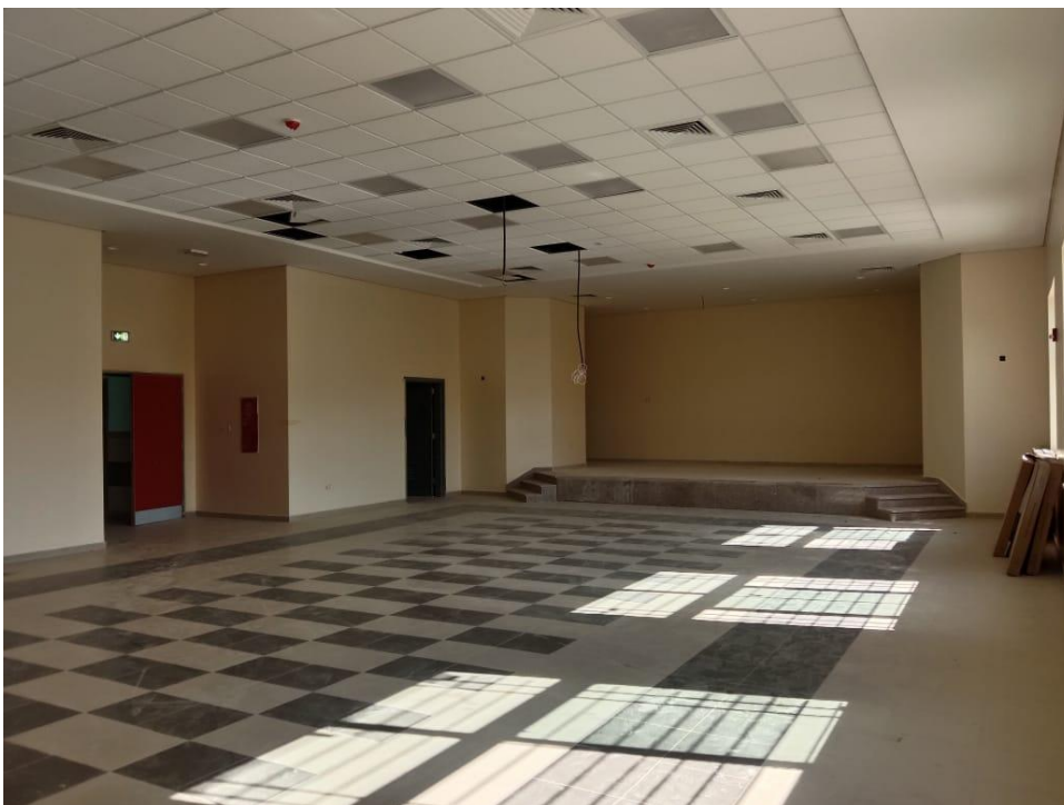
Works at the multi-purpose hall
