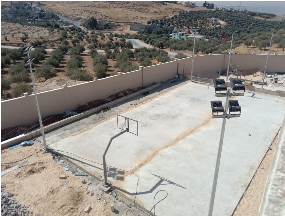
External works at the playground and the parking area
