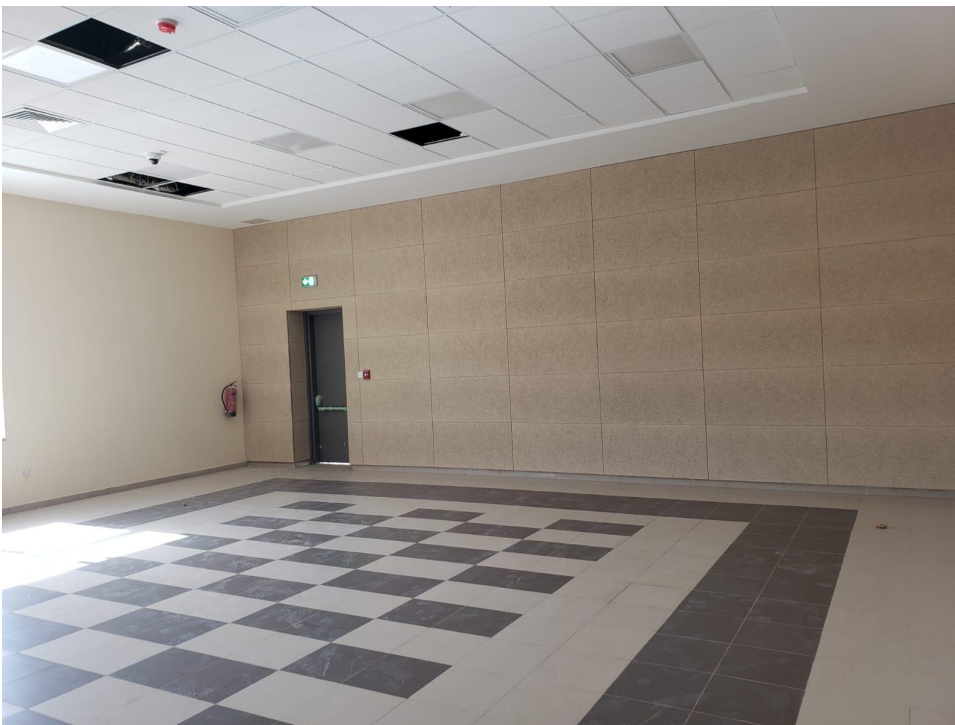
Finishing the Hera Design works at the multi-purpose hall
