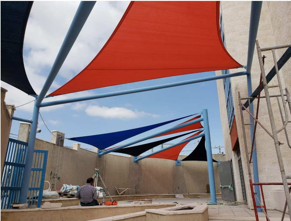
Installing tensile shadings at the KG entrance
