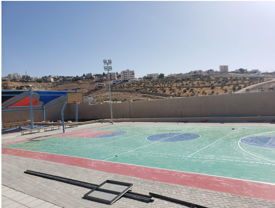
Painting work for the playground
