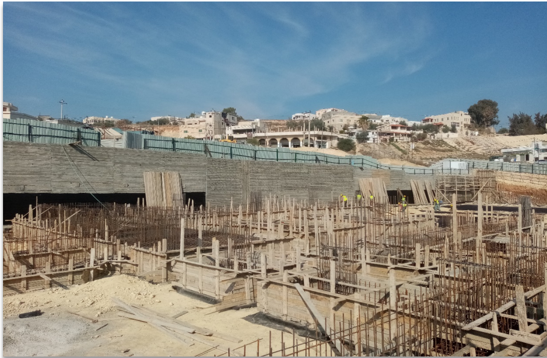
Figure 3: Reinforcement Steel Laying and Frameworks in the Southern Section
