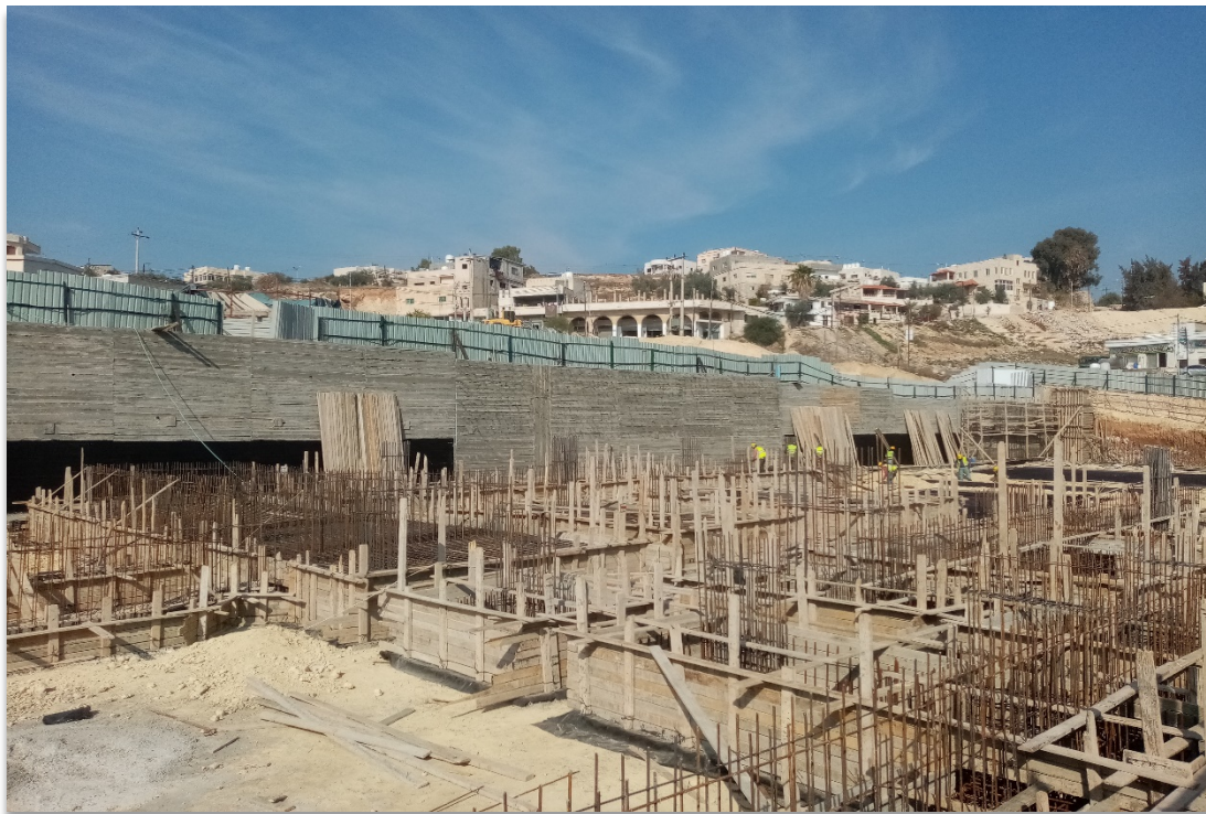
Figure 2: Overview of the Southern side of the Construction Site
