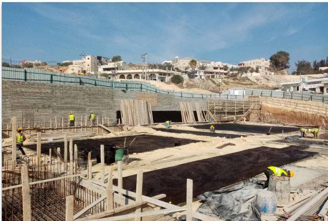
Figure 4: Blinding Insulation in the Northern Section
