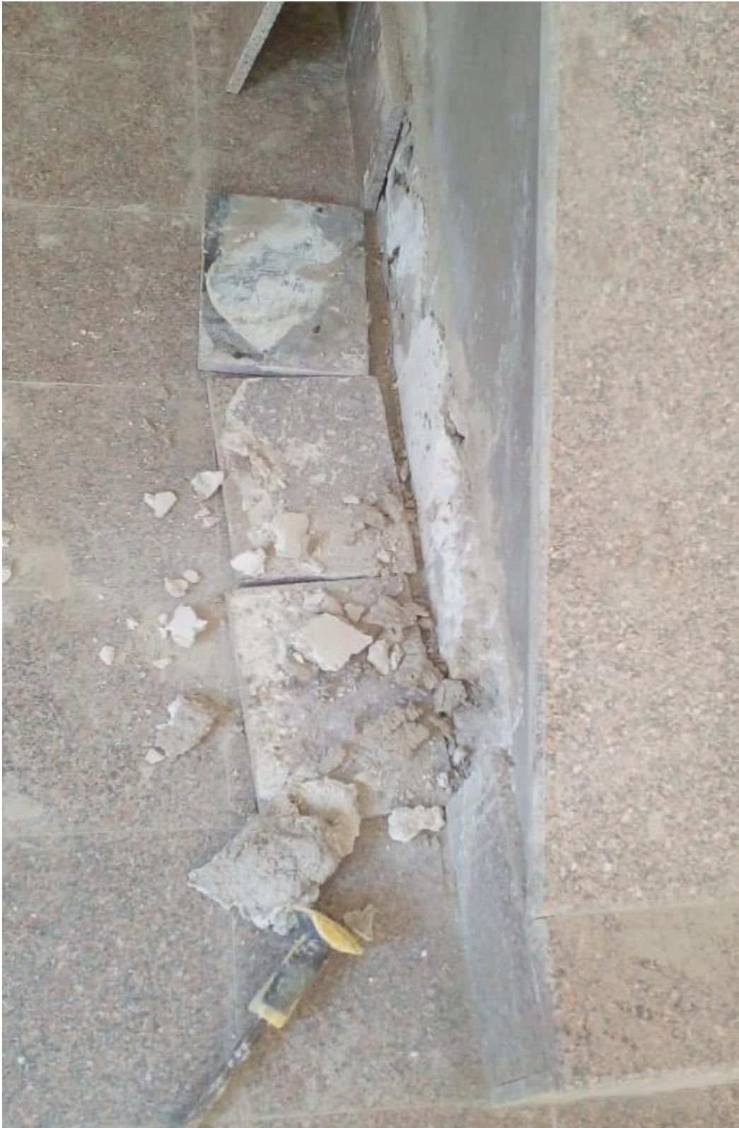
Replacing the granite at staircase due to the black spots
