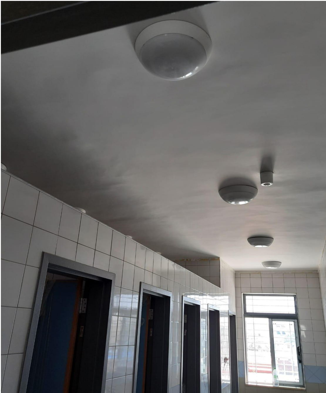
Waving in the plastering/painting of the ceilings of toilets
