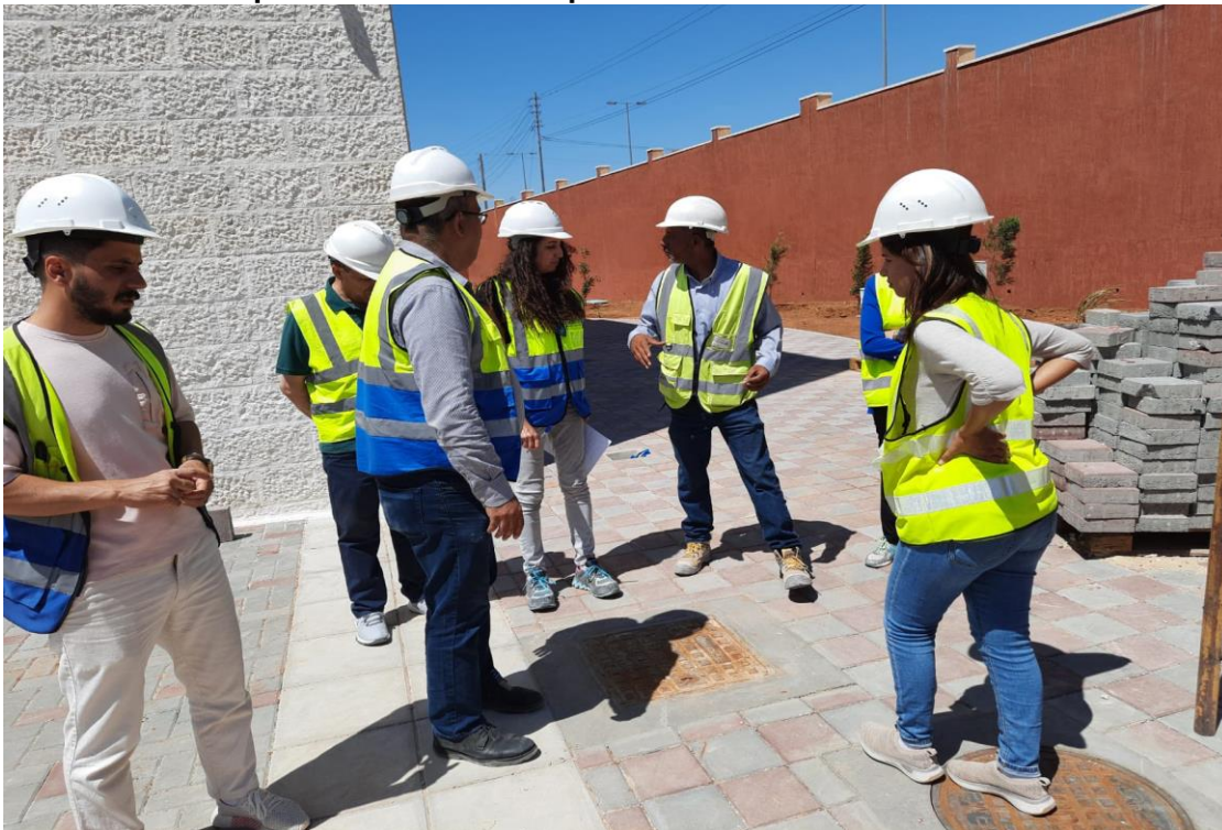
Manholes covers need cleaning from corrosion, and paint
