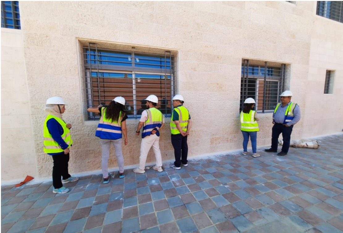
Parts of the steel protection screens are painted with different color
