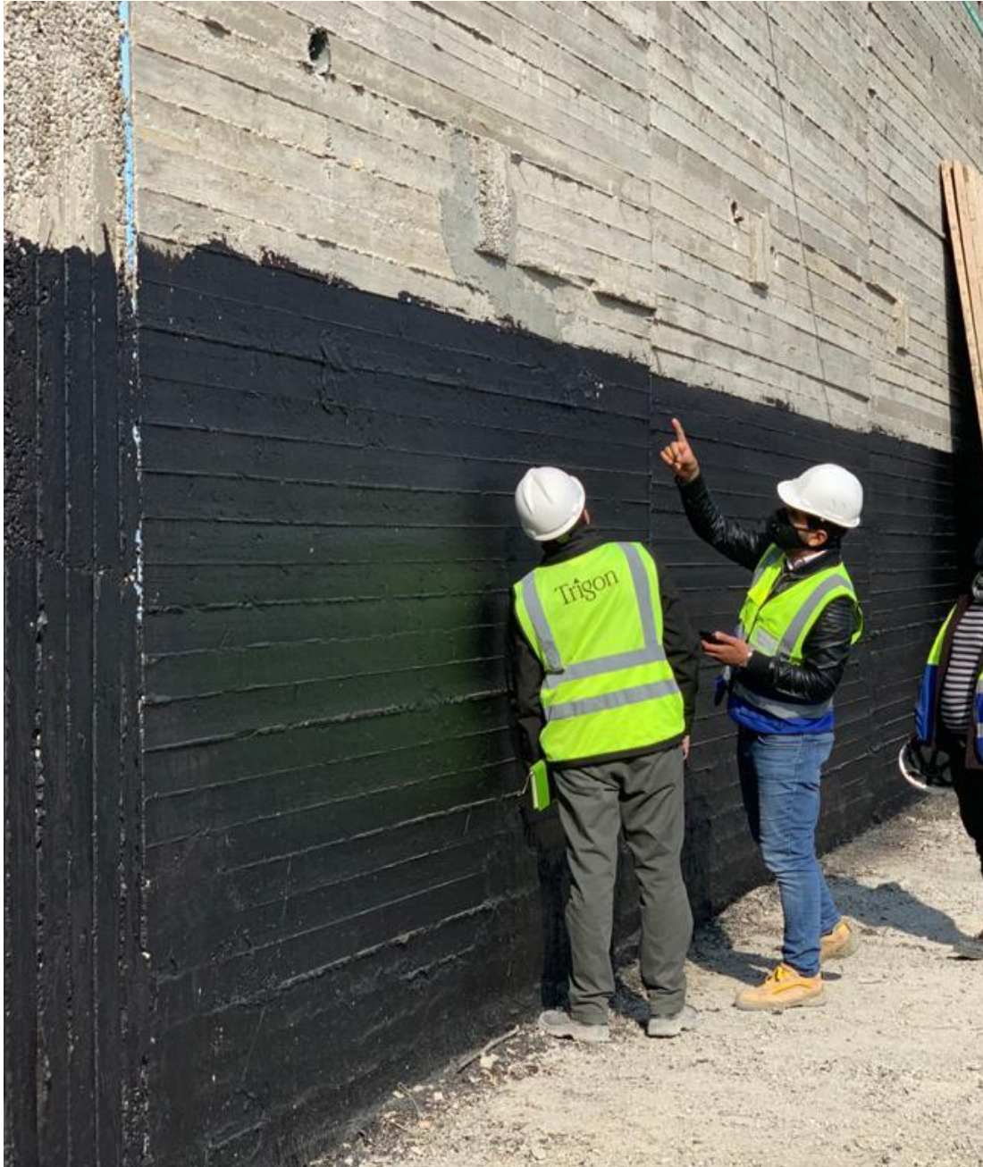
Watching wall insulation
