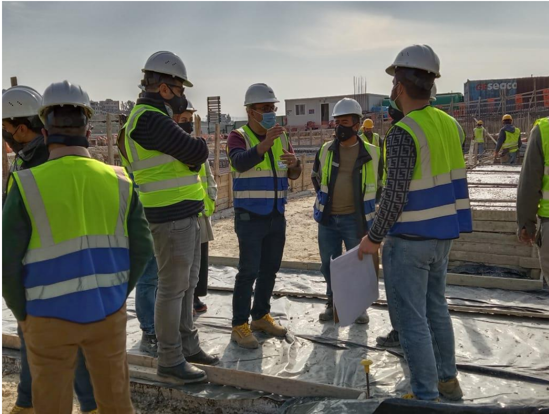
Eng. Natheer discussing work progress on site
