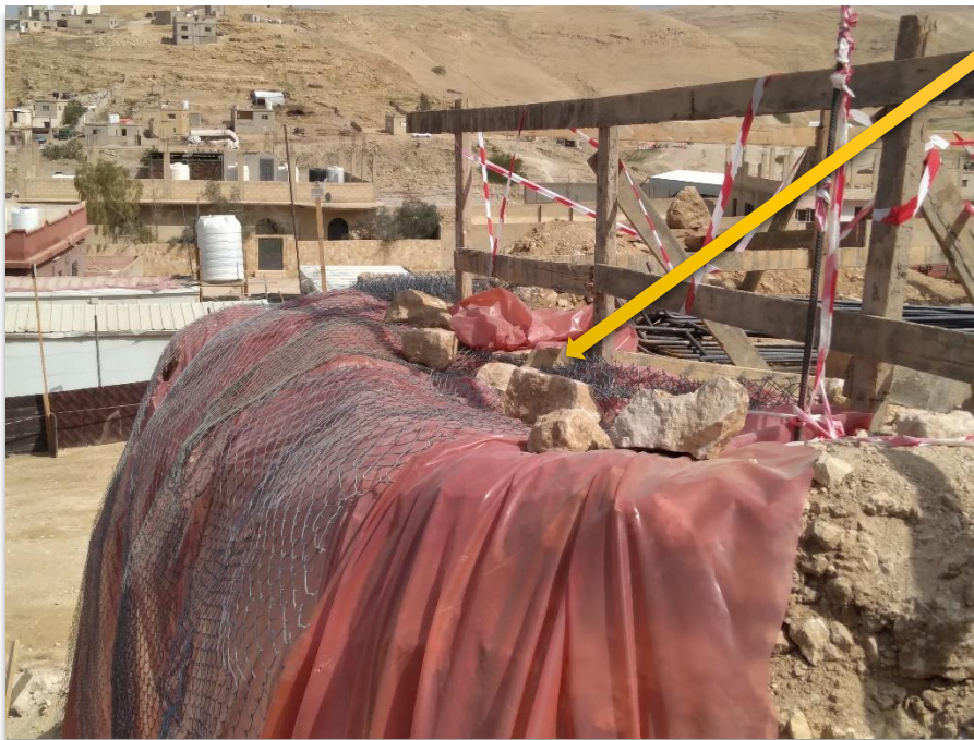
Figure 11: Falling Object Hazards
