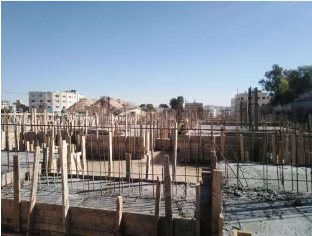
FIGURE #10 & 11: New construction building will consist four floors and roof (basement, ground floor, first floor and second floor). The total area is 5700 sq.m and external area is 5600 sq.m including Basketball Court works Construction of building's foundation is completed
