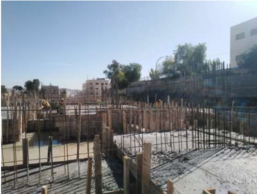
FIGURE #06 & 07: New construction building will consist four floors and roof (basement, ground floor, first floor and second floor). The total area is 5700 sq.m and external area is 5600 sq.m including Basketball Court works Construction of building's foundation is completed
