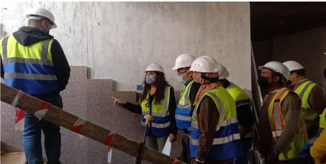
Defects in granite cladding for staircase
