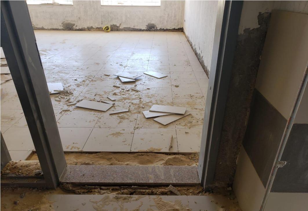
Replacing of defected threshold
