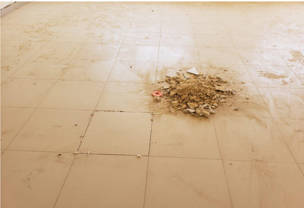
Replacing of defected floor tiles
