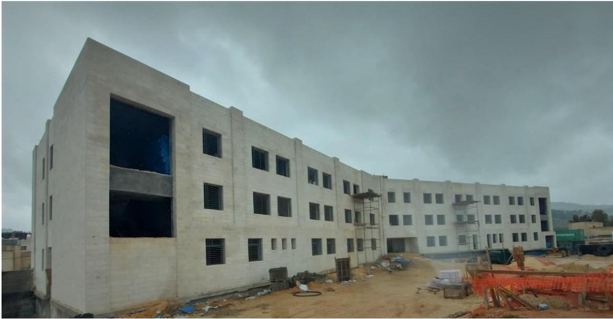
General view of the project site
