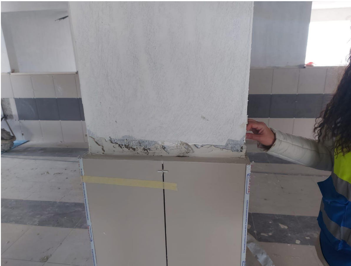
Inspecting porcelain column cladding at the corridor
