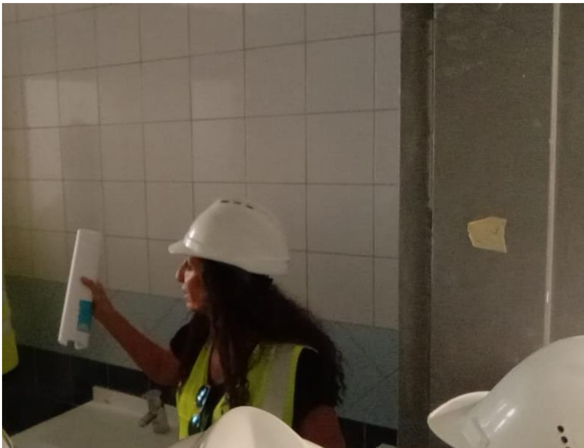
Checking tiling work at the wet areas
