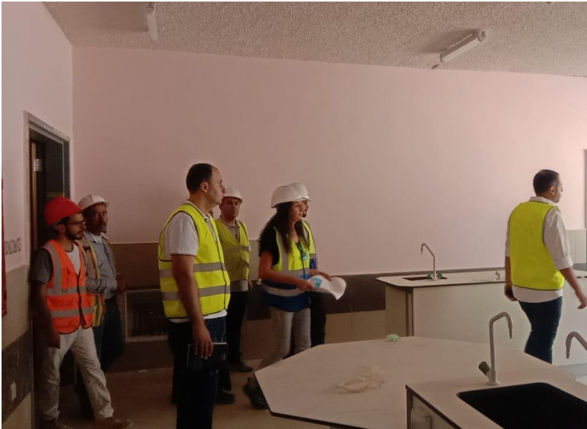
Inspecting laboratories furniture installation and electro-mechanical connections
