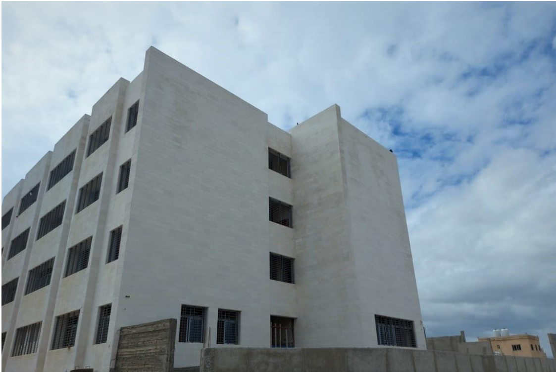
General view of the project site
