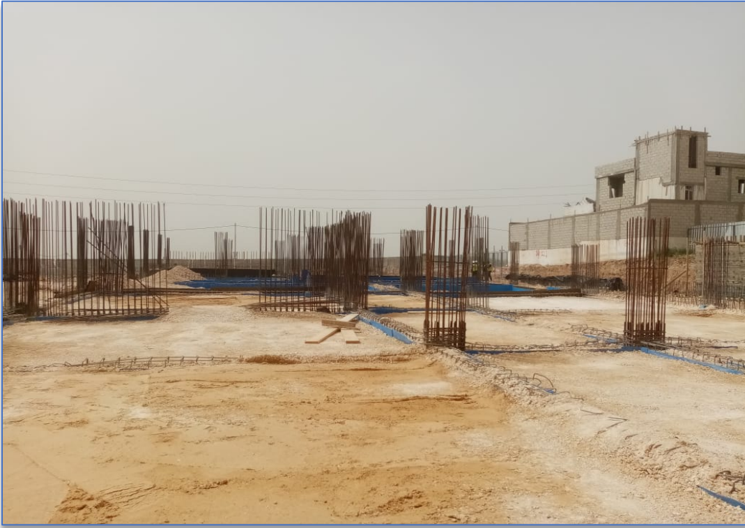
Figure 3: Slab on Grade Preparation
