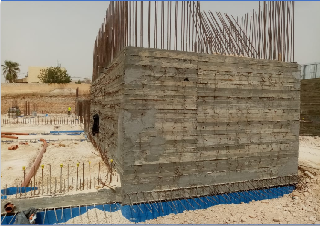
Figure 5 Segregation in Staircase walls
