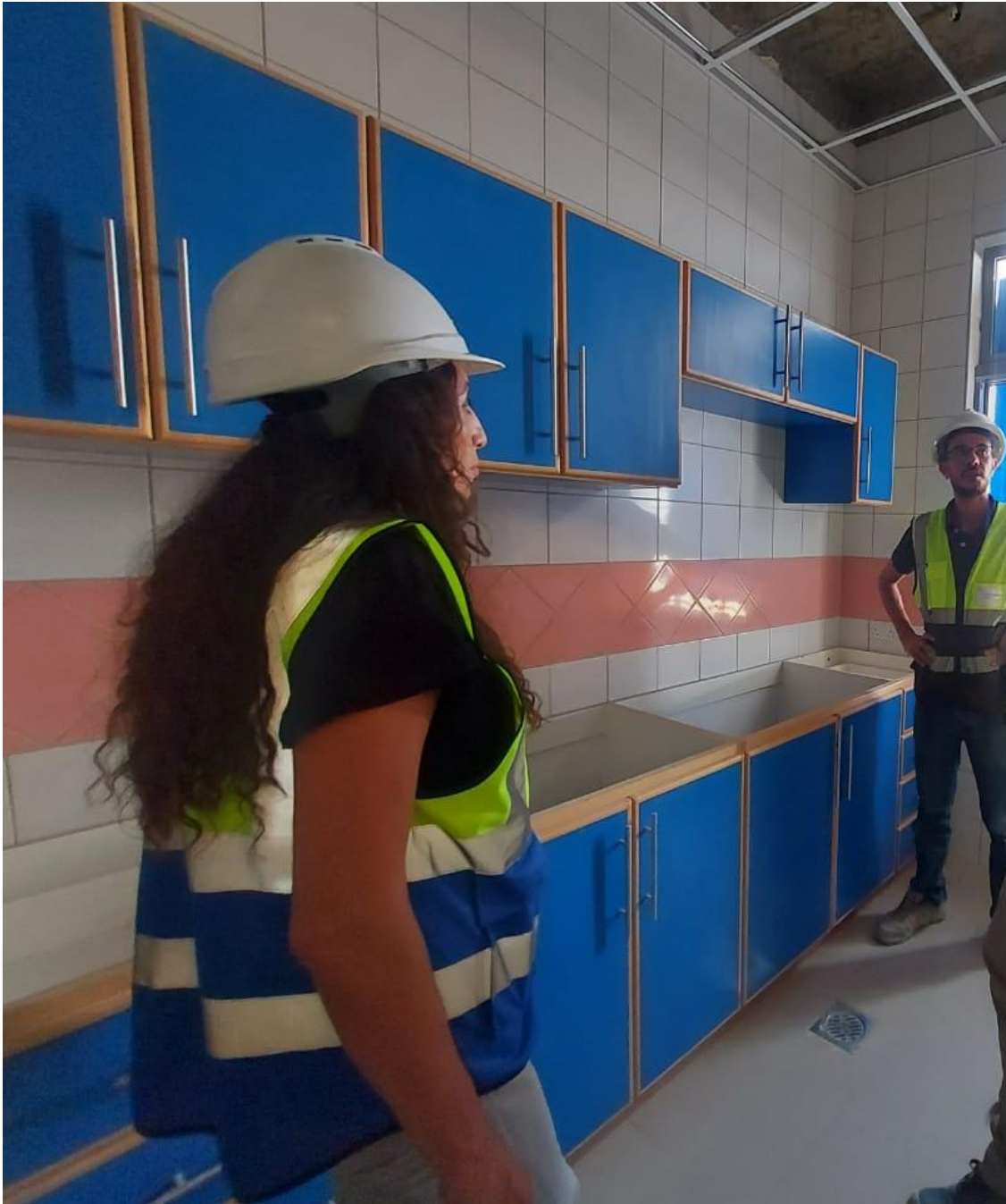
Observing cabinets re-installation after rectification
