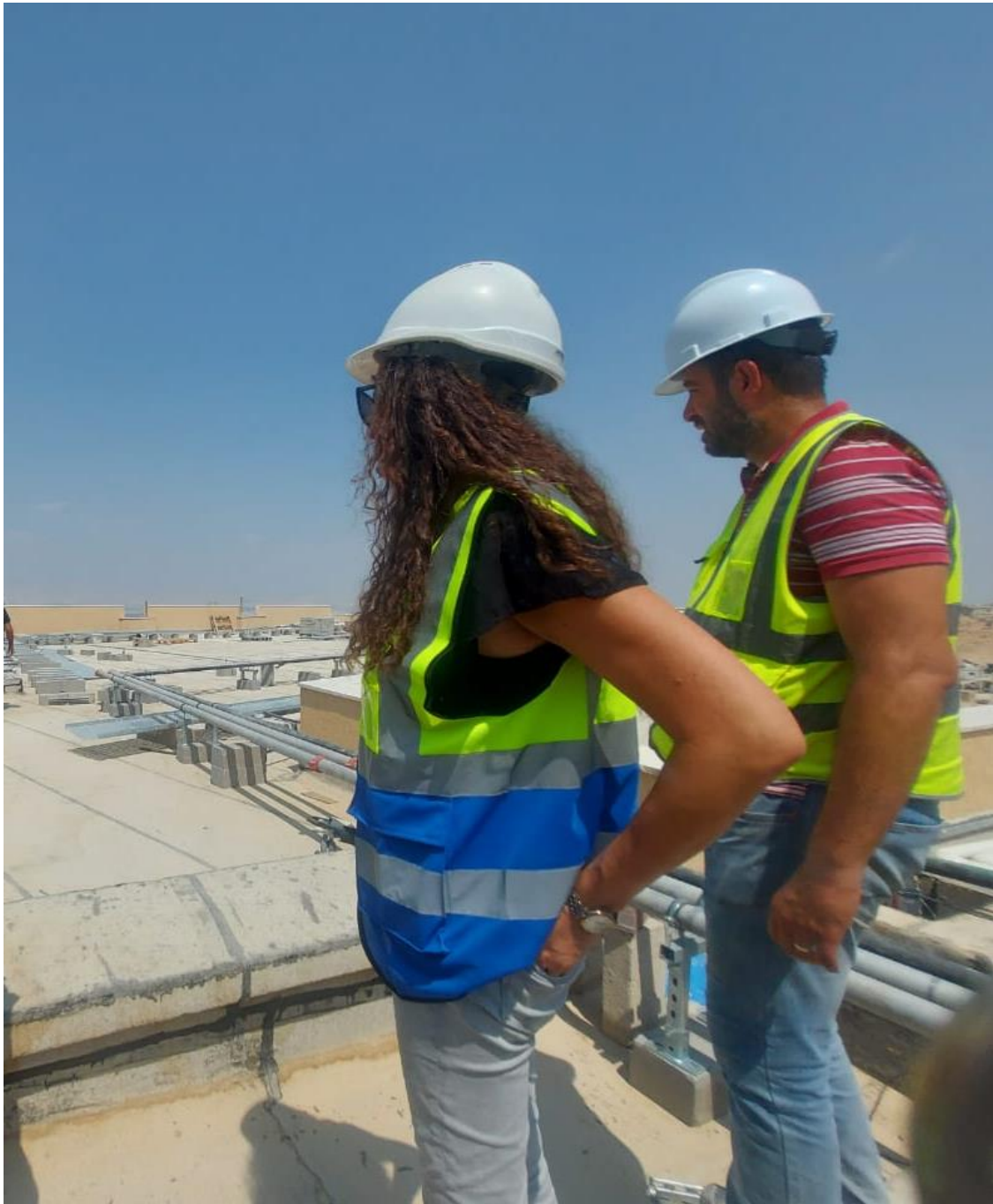
Inspecting executed works at the roof
