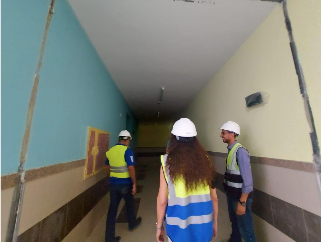
Observing works at the corridors
