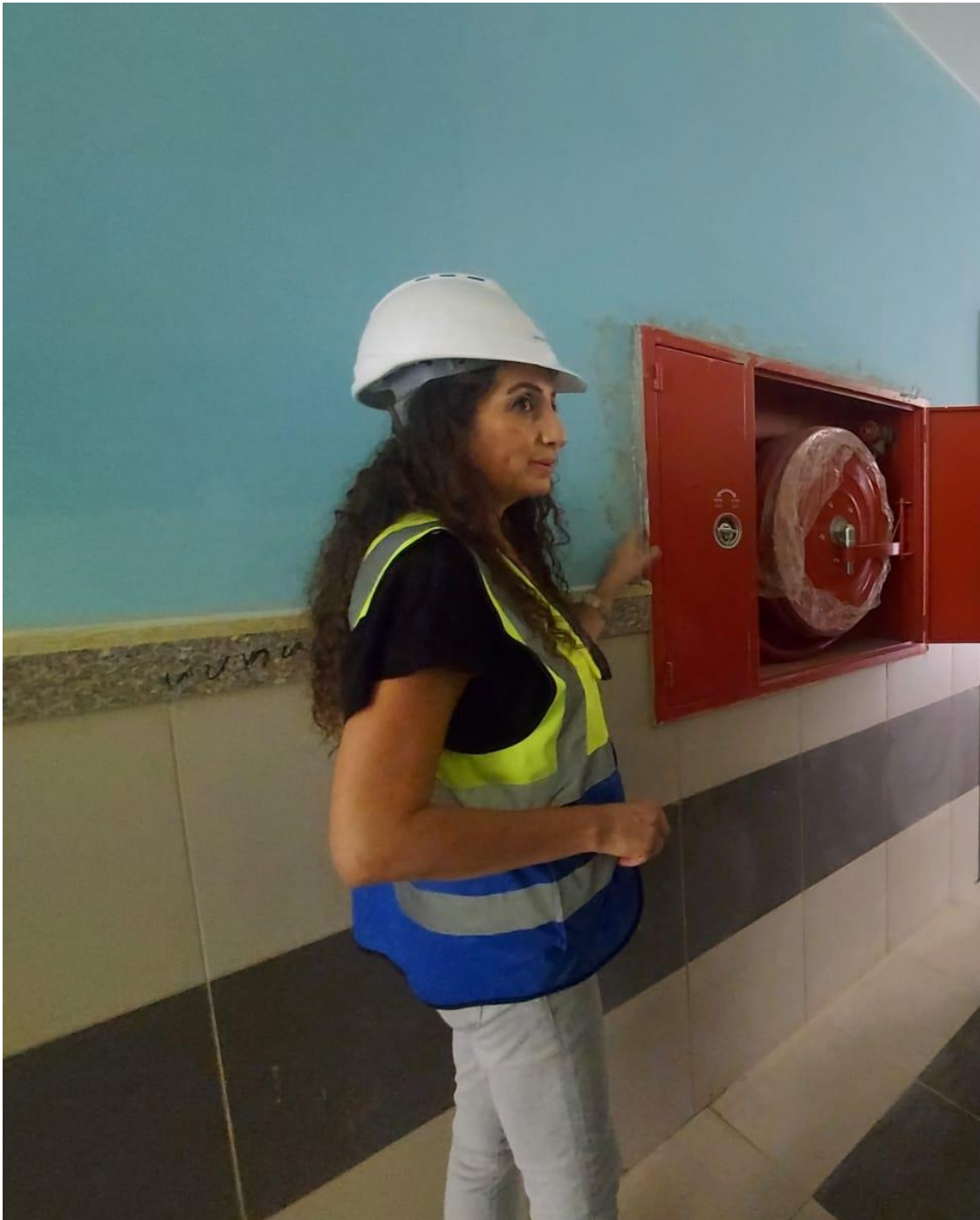
Inspecting fire hose cabinets at the corridors
