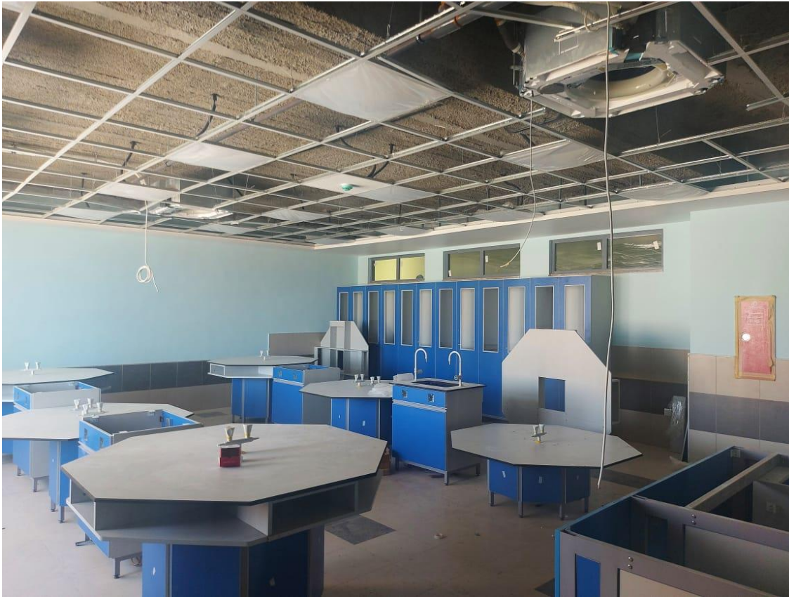
The team inspected the installation of lab furniture
