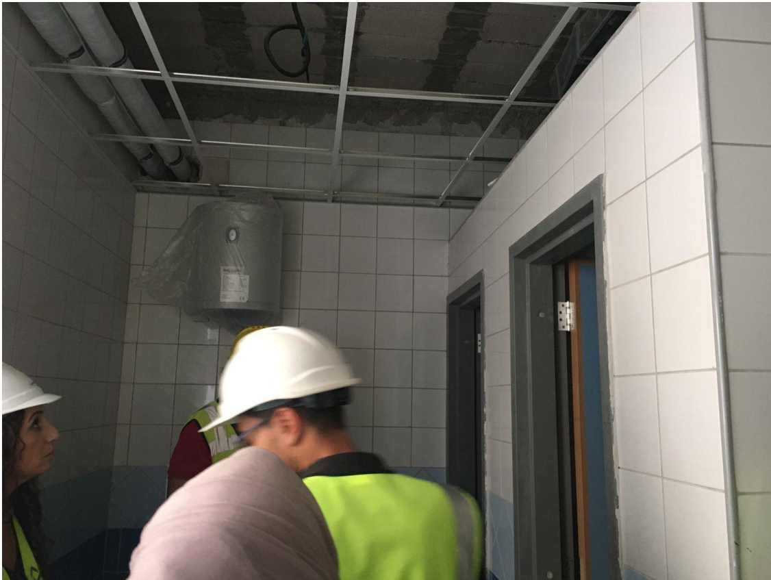
Checking the installation of heating pipes at the wet areas
