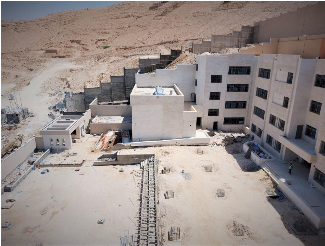
General view of the project site
