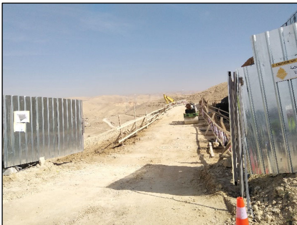
Figure #3: GATE (2) – Site Equipment & Vehicles Entrance. Photo credit: Odai Tawalbeh, 1/25/2021
