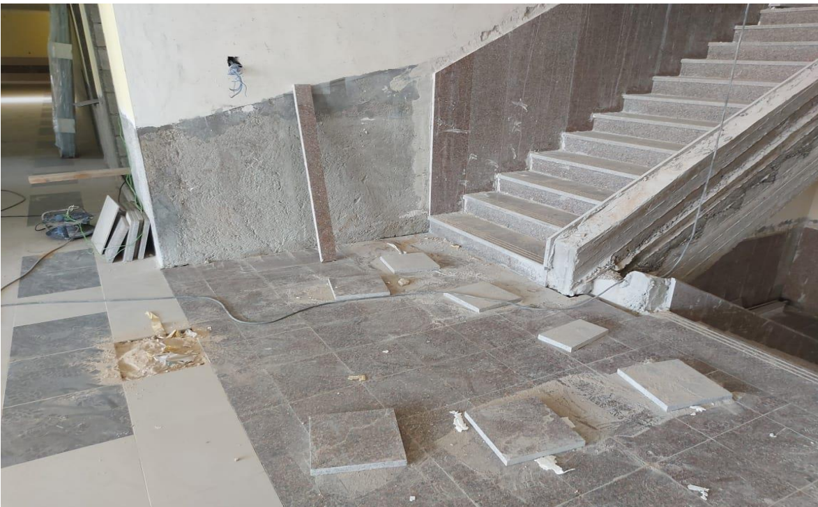
Re-tiling complying with the workshop drawings
