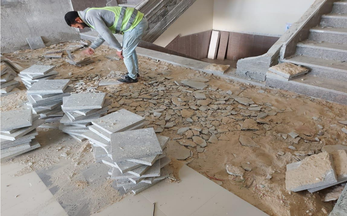
Removal of the granite tiling
