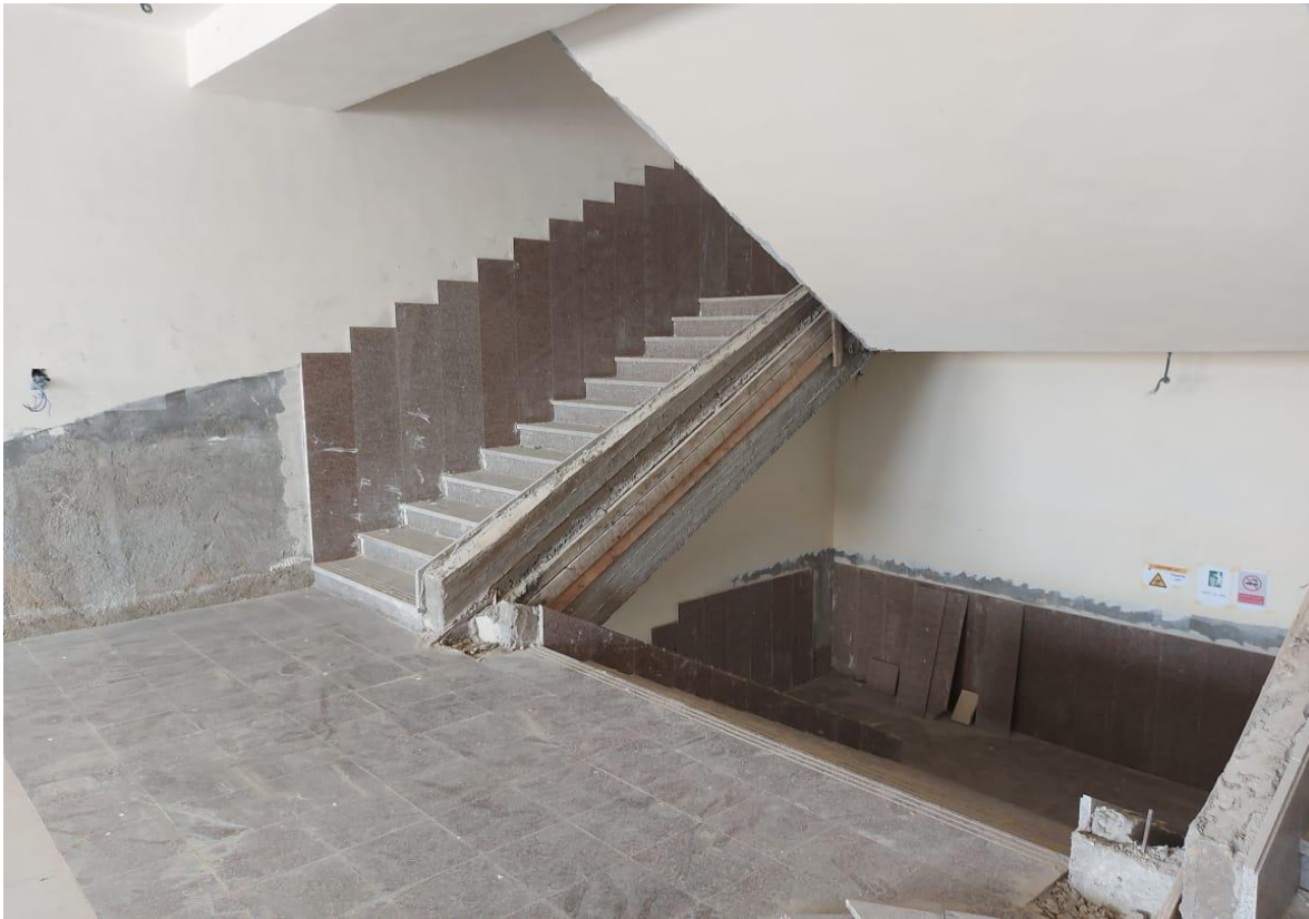
Completion of re-tiling
