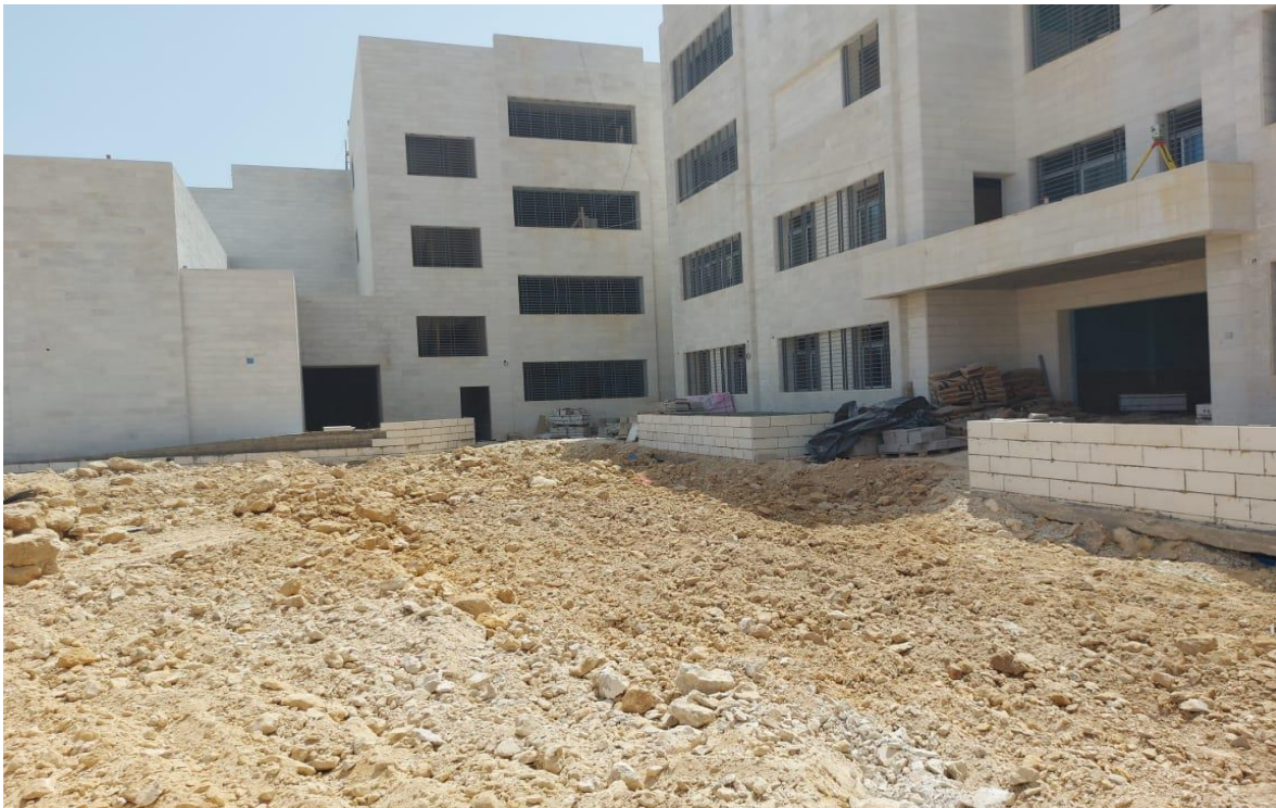
Dirt at the stone facades
