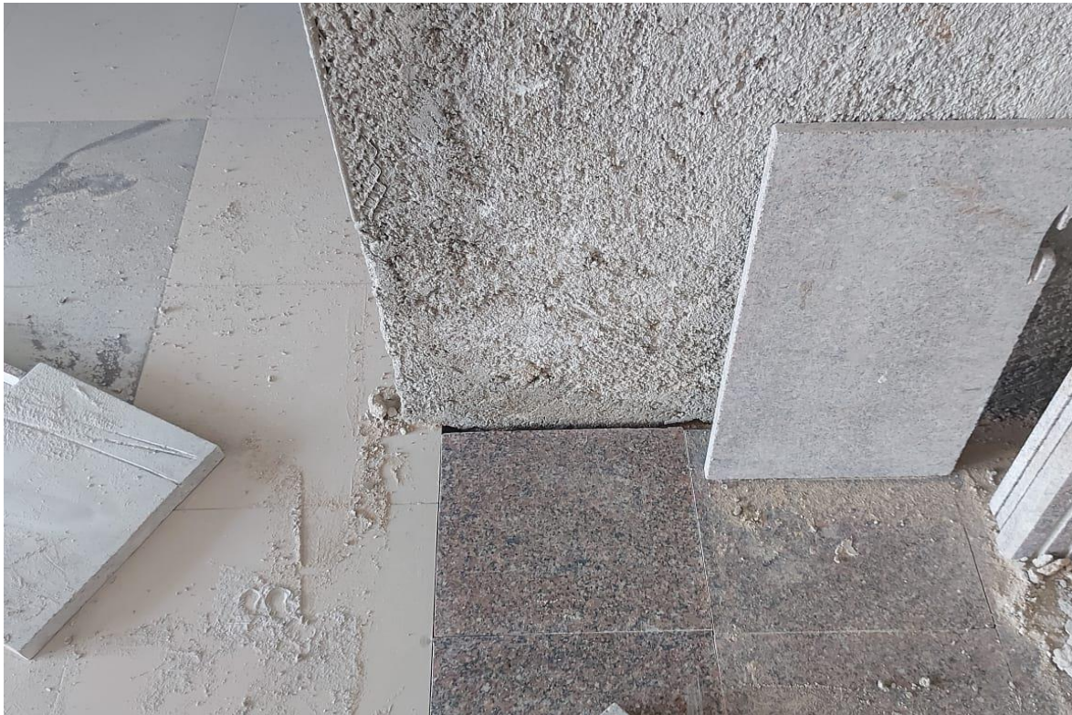
Tiling not complying with workshop drawings
