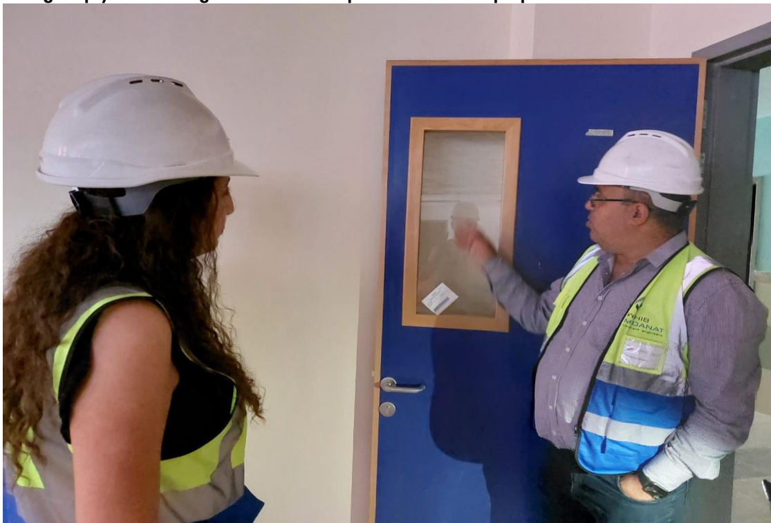
Dimensions of the vision panel of the wooden doors are less than specified
