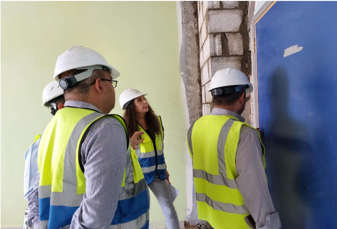
Defects in the cutting of laminated sheet and beech wood frame of the doors
