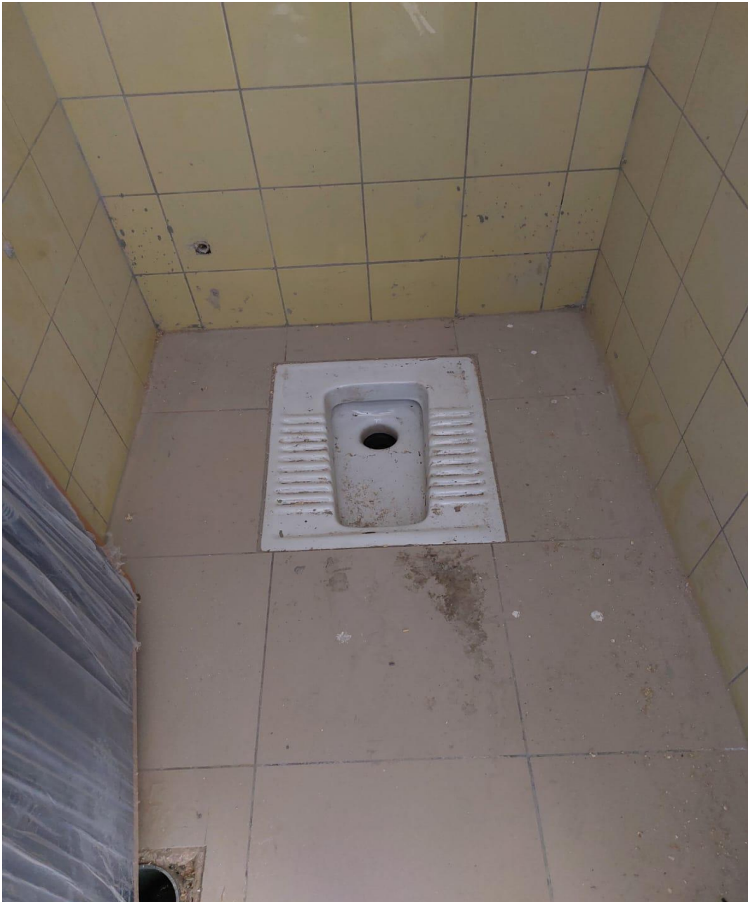
Removal of debris and dirt from sanitary fixtures
