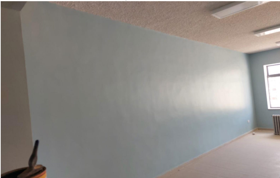
Waving in plastering
