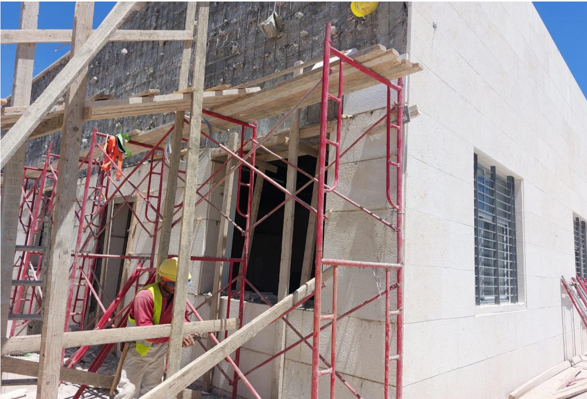
Rebuilding of stones
