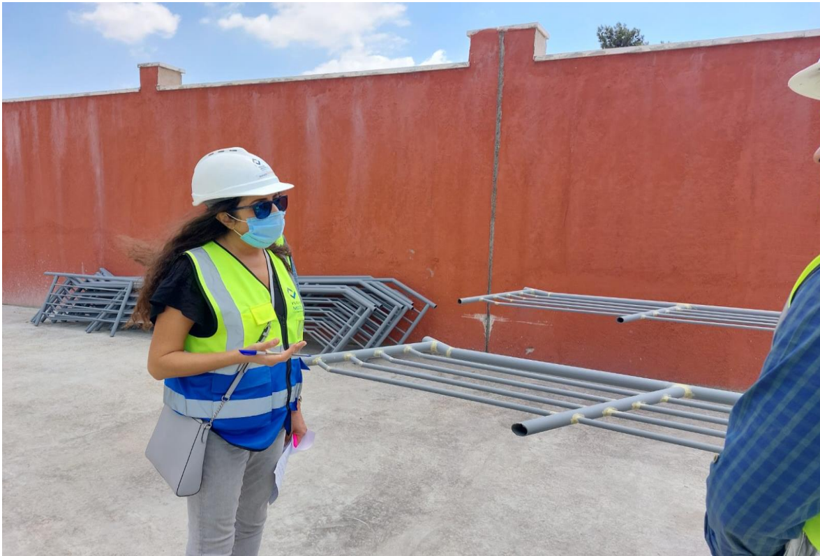
Defects in the handrails and dirt at the boundary walls
