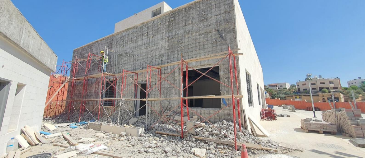
Removing defected stones
