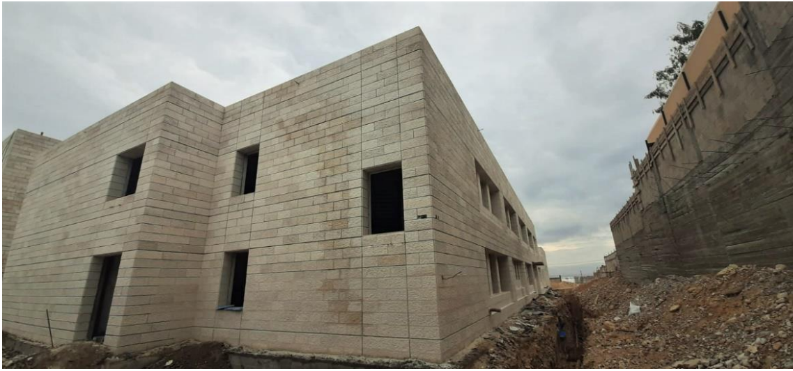
General view of the project (Figures: 01, 02 & 03)
