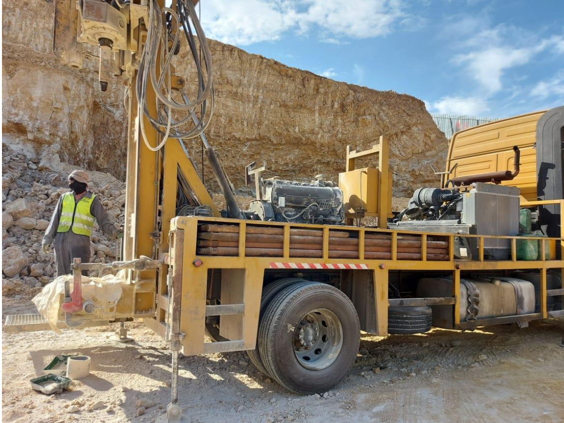
Boreholes excavation by the specialist's laboratory
