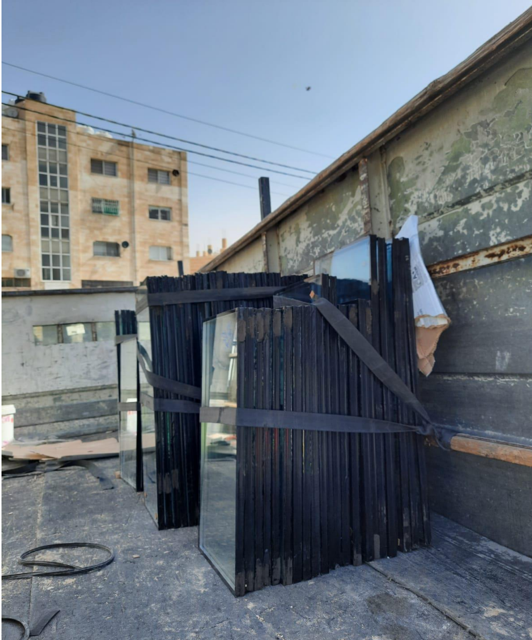
Dismantling of defected aluminum sections
