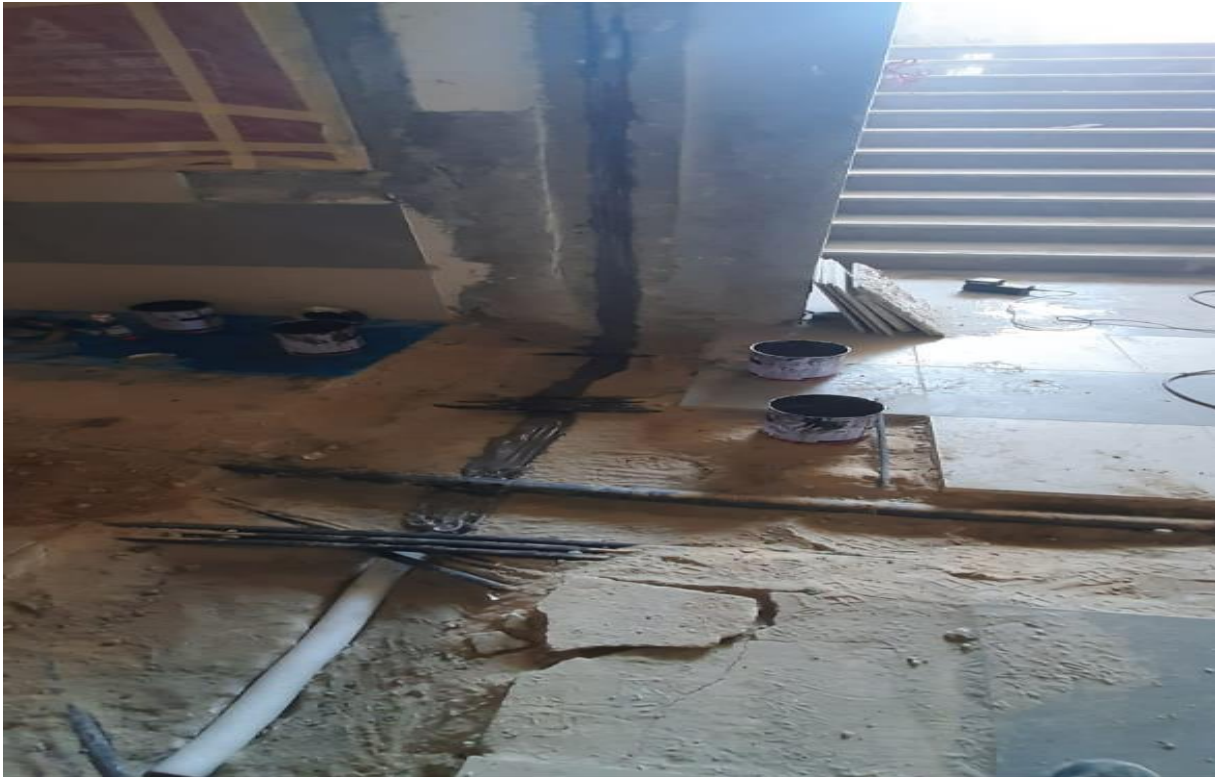
Reducing the level of electrical conduit
