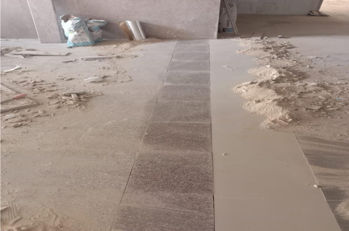
Rectification of granite and porcelain tiles to match
