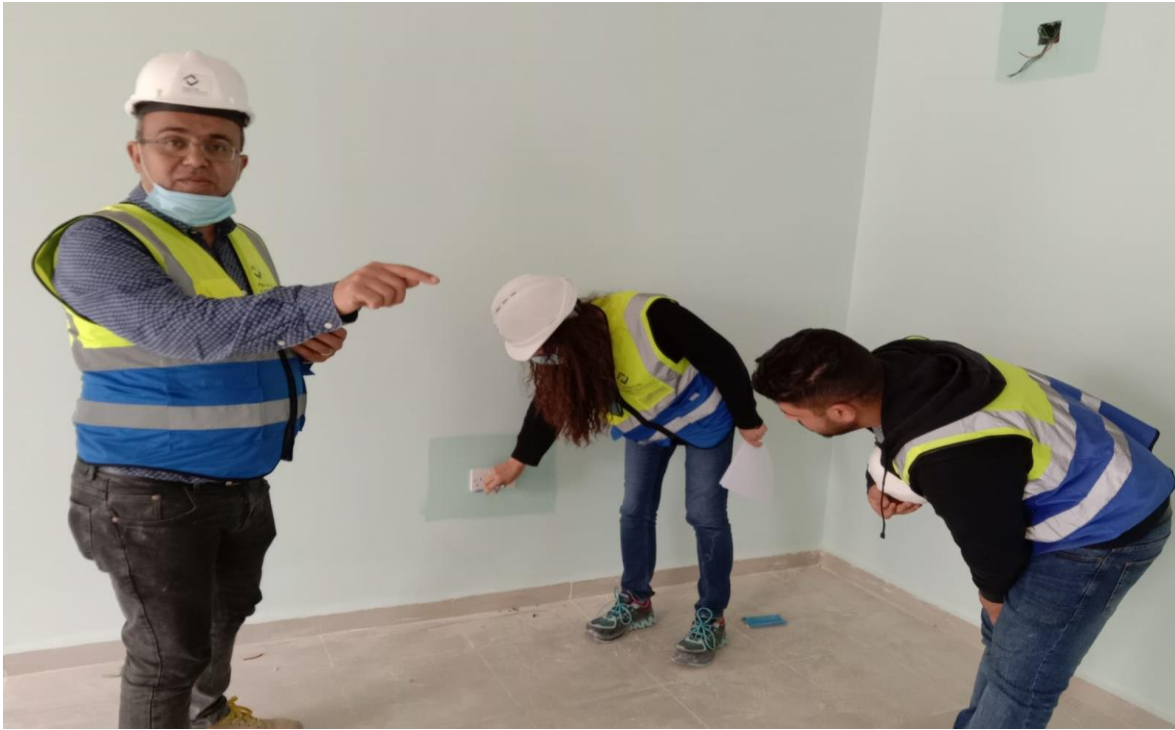
Fixing sockets before completing the paint work
