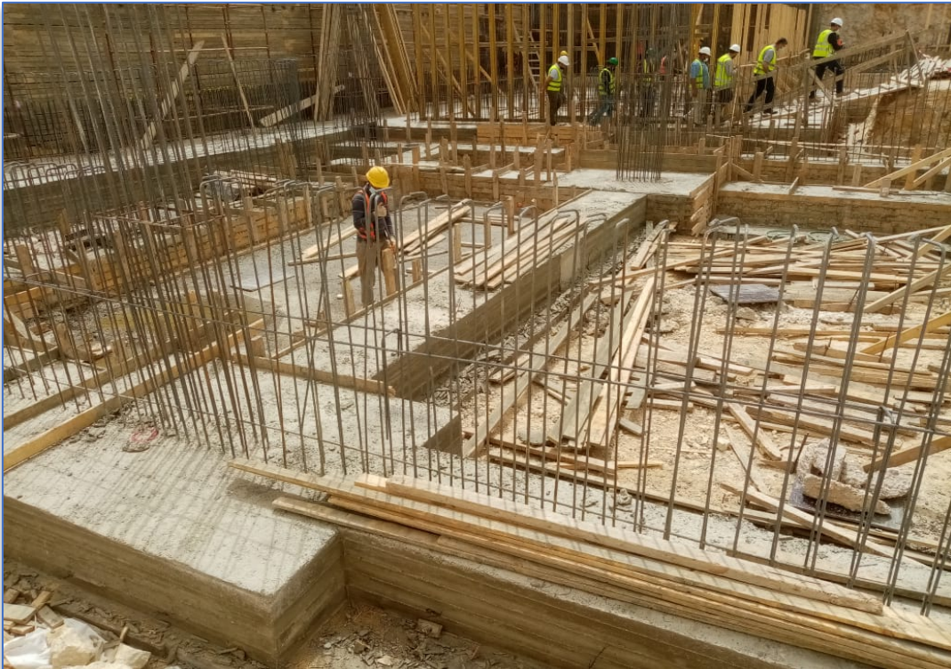
Figure 6: Dismantling Formwork
