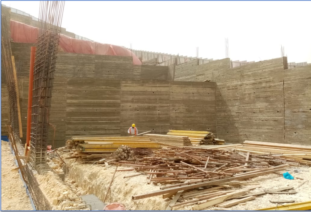
Figure 5: Finished Retaining & External walls
