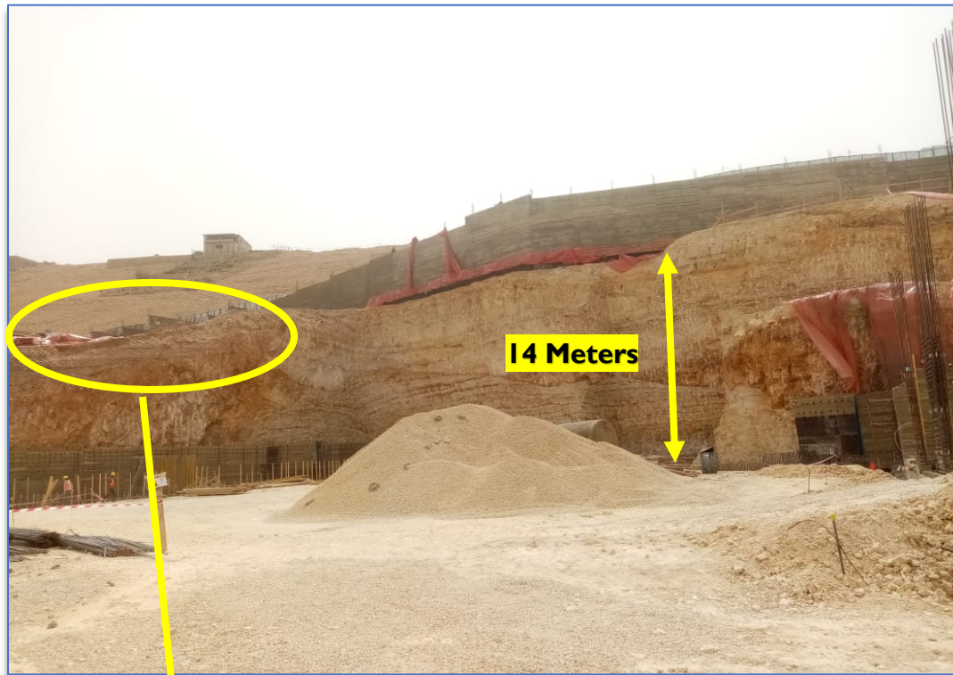
Figure 3: External Boundary Wall and proposed Shoring System
