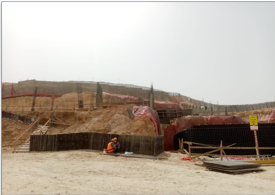
Figure 1&2: Southern view of the Construction Site
