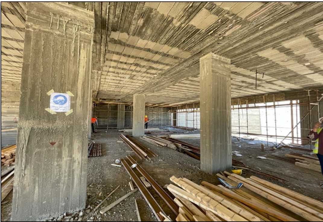
Figure 4: Framework de-shuttered and preparing for Block works
