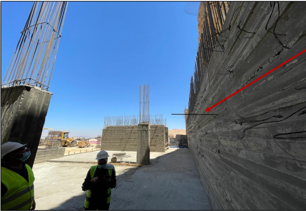
Figure 9: Protruding Reinforcing Steel
