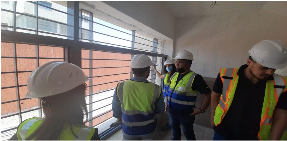
Defects in the steel protection screens
