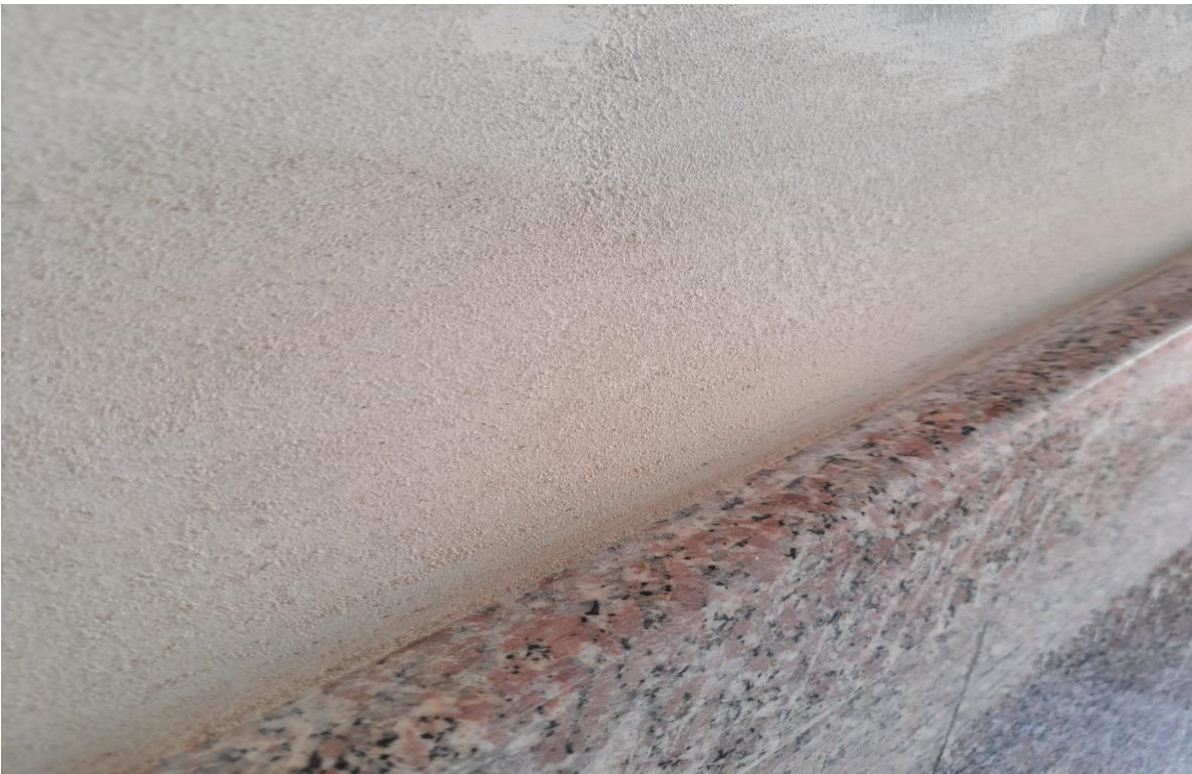
Rectification of installed granite coping
