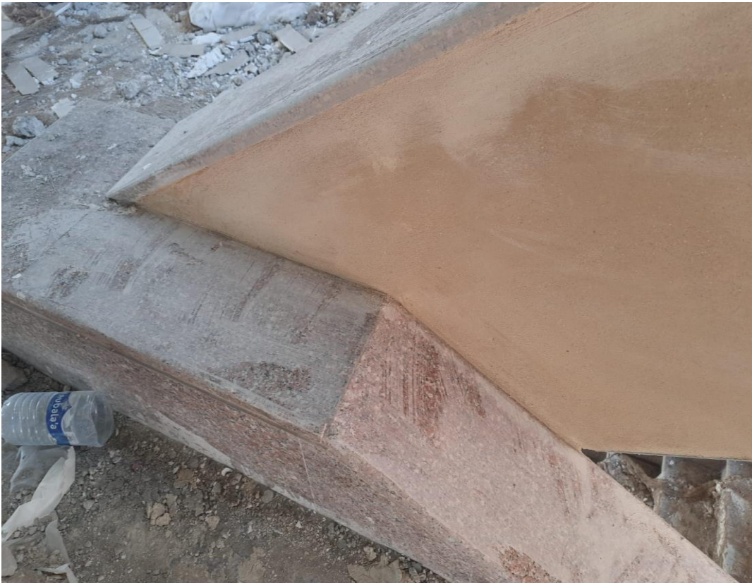
Rectified granite tiling
