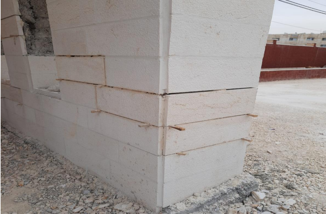
Replacing defected stones at the guard house
