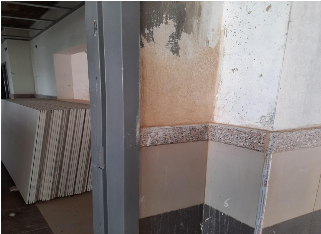
Rectified granite coping
