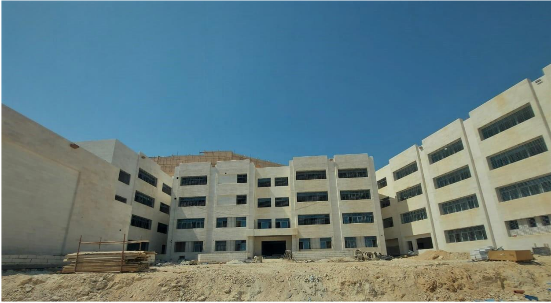
General view of the project site
