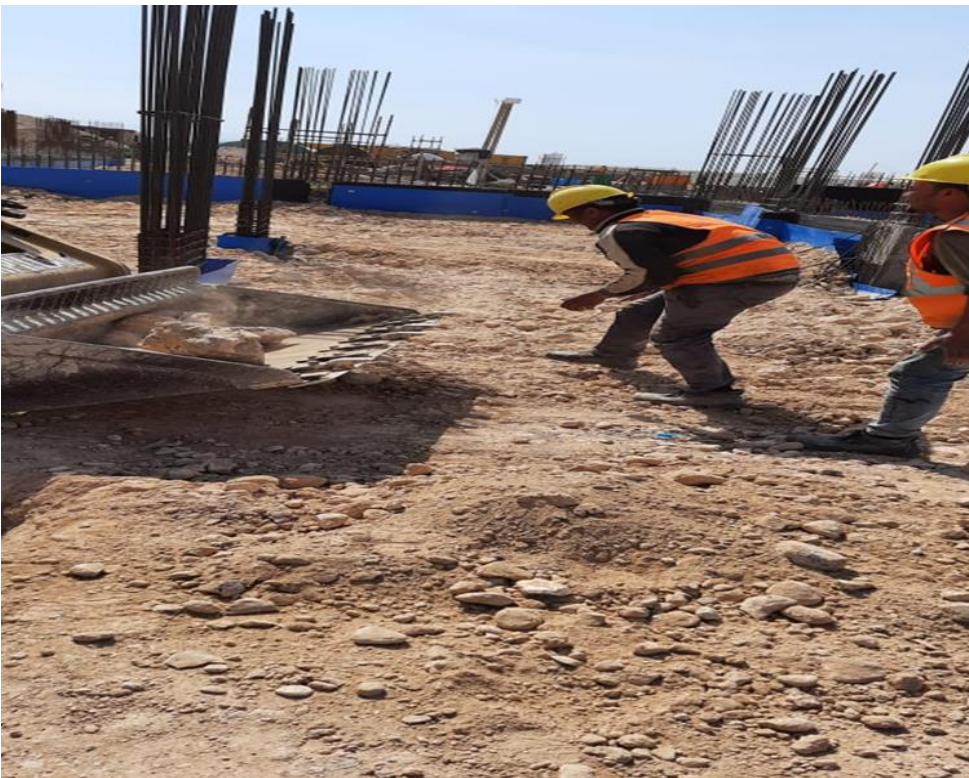
Removal of Boulders- QC Report 1301
