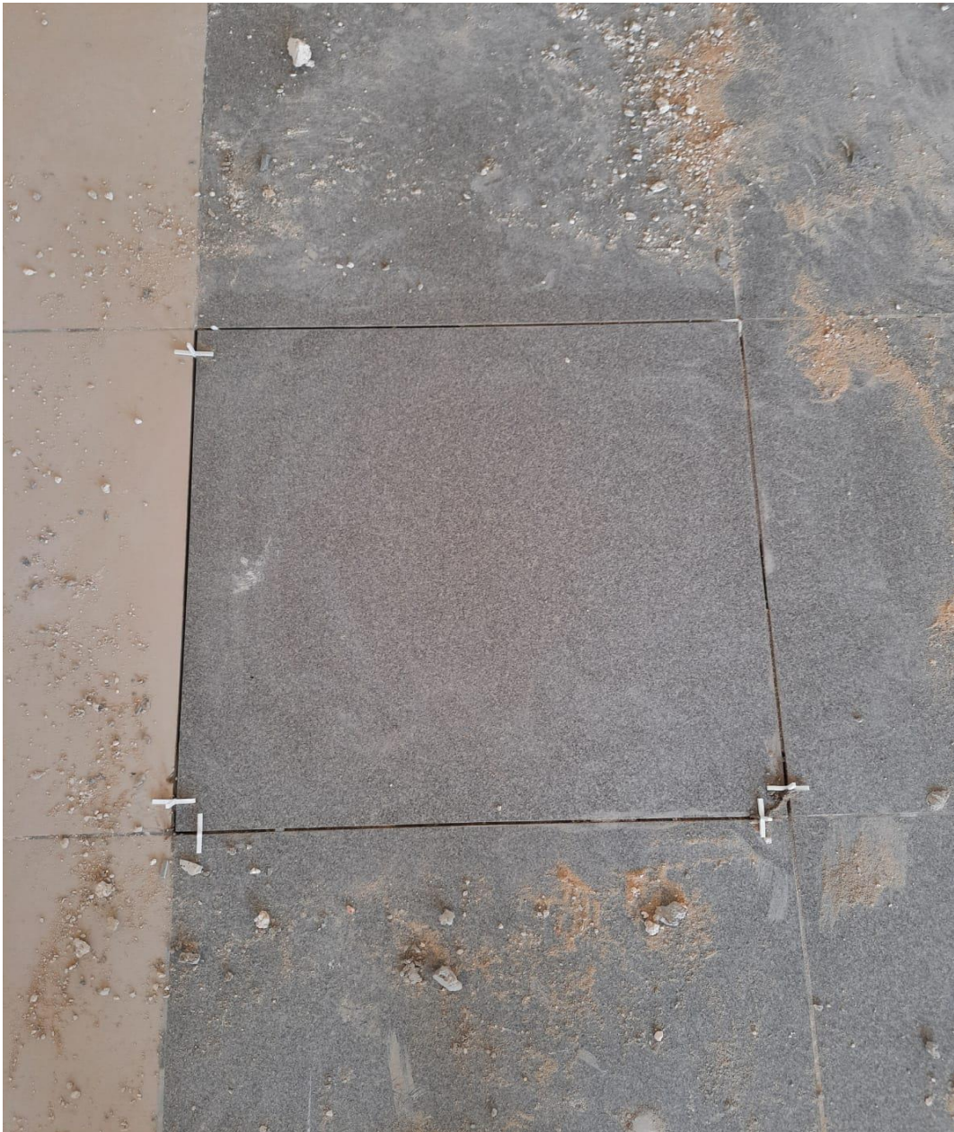
Replacement of defected tiles
