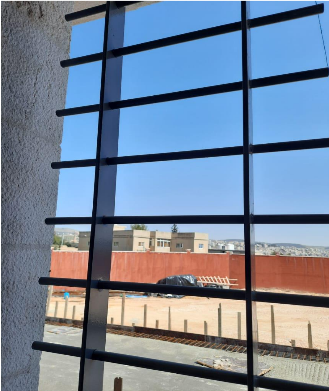
Rectified steel protection screens
