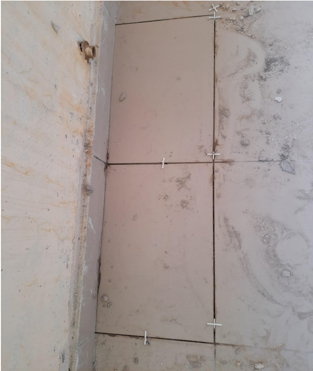
Replacement of defected tiles
