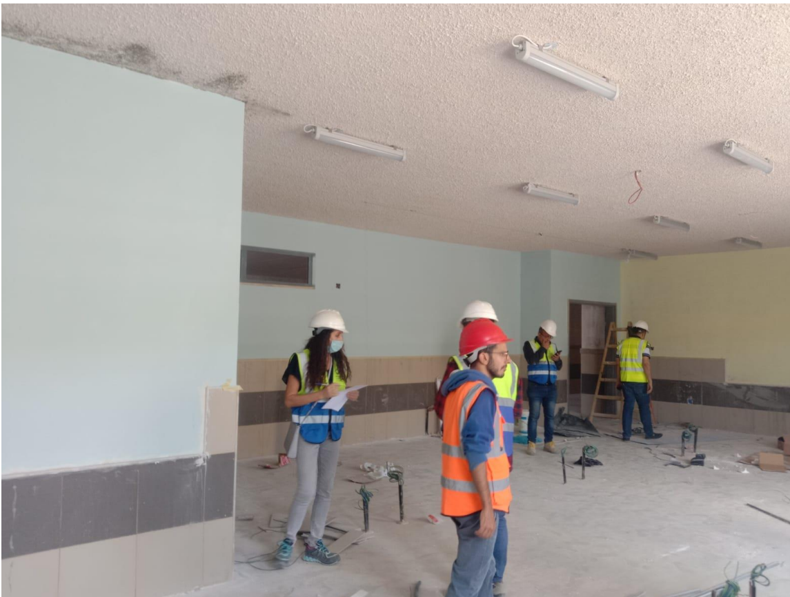
The team inspected the executed works at the art room
