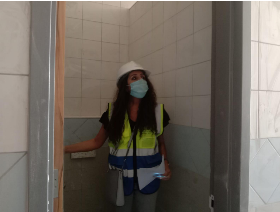
The team inspected tiling work at the wet area
