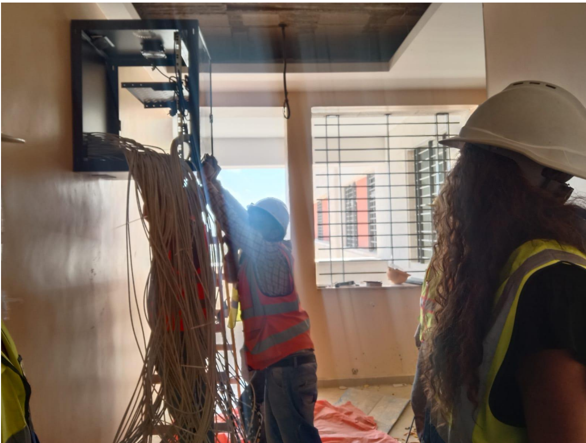
Installing the data cabinet
