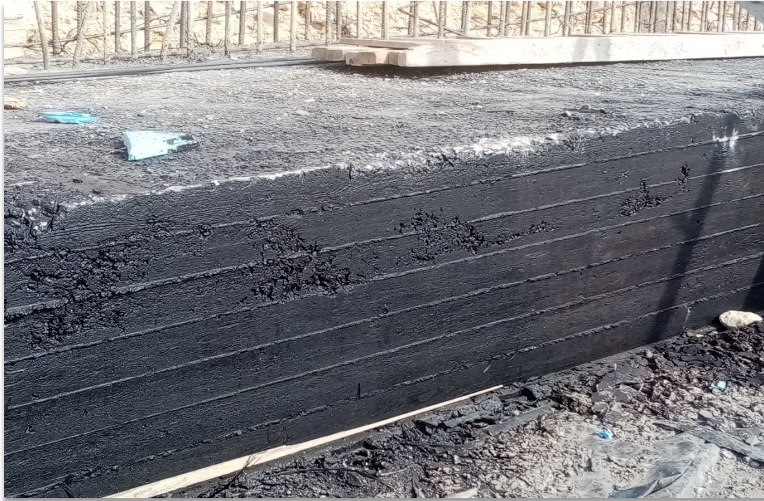
Figure 7: Bitumen Insulation
