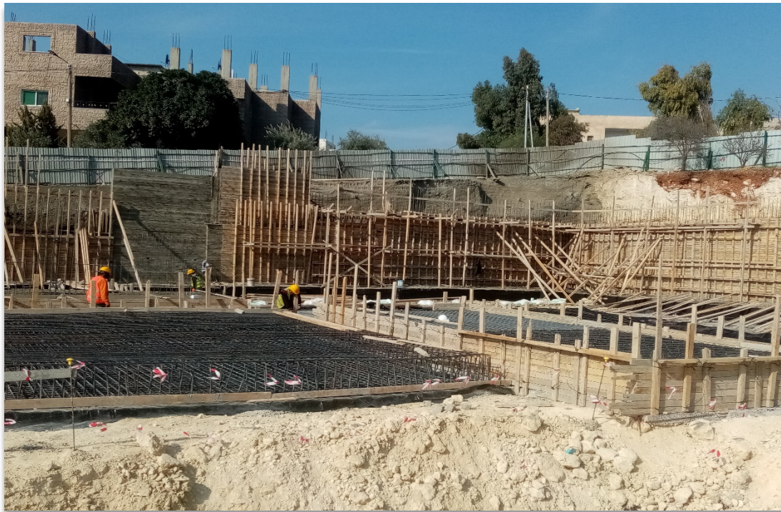
Figure 3: Construction Contractor De-Shuttering Retaining Wall Framework
