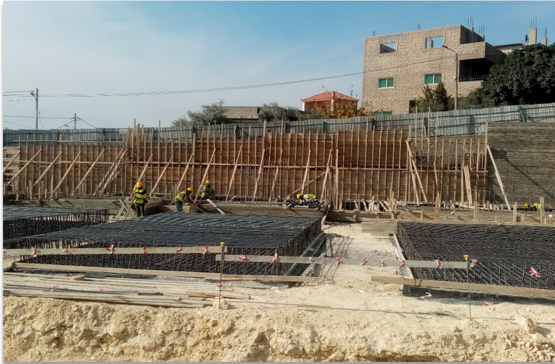
Figure 3: Construction Contractor De-Shuttering Retaining Wall Framework
