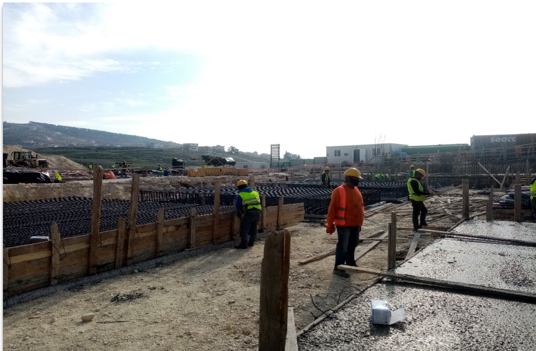
Figure 2: Overview of the Construction Site
