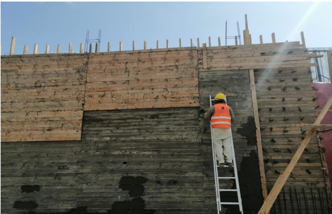
Repair of Segregation- QC Report 1304
