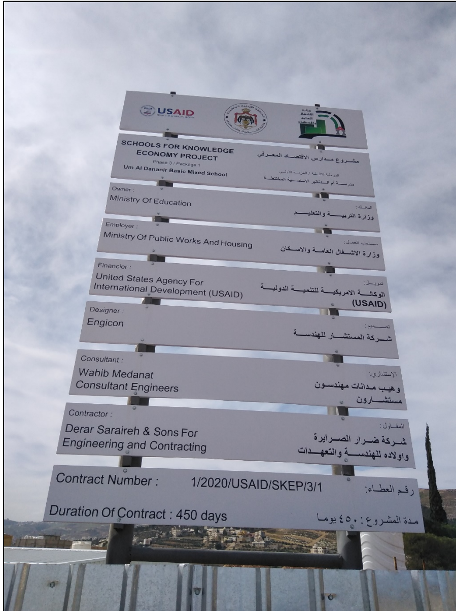
Figure #1: Project ID Sign Board on site.
