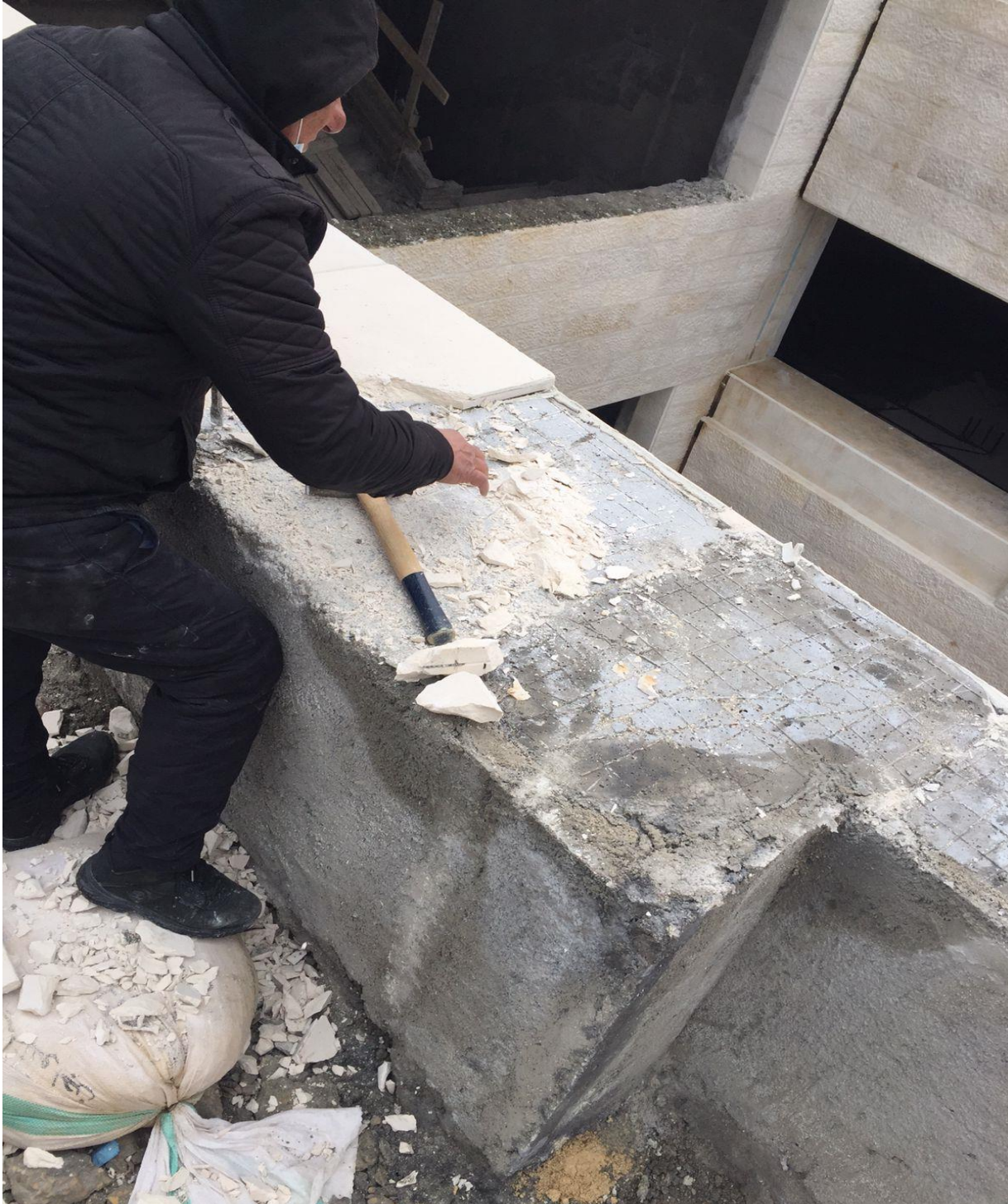
Removal of defected stone coping
