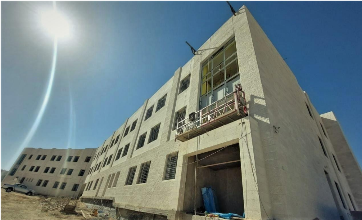
General view of the project site
