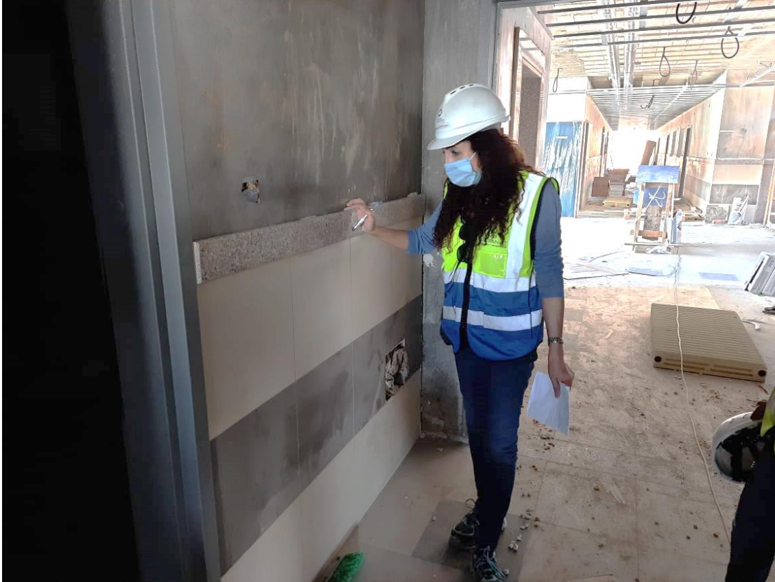
The team inspected the installed porcelain wall tiles at the corridors
