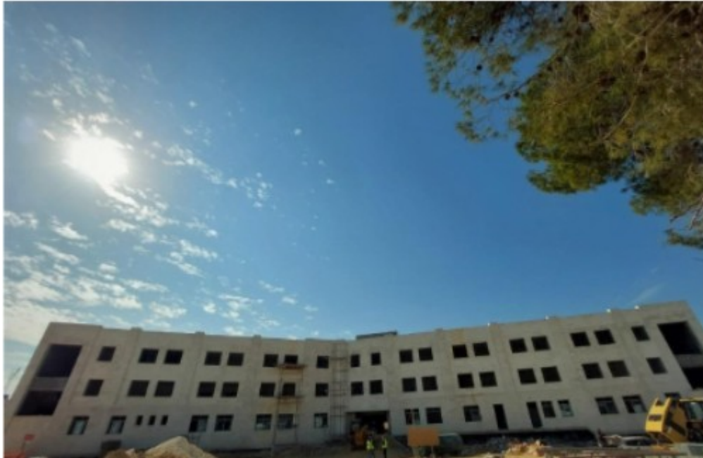
General view of the project site
