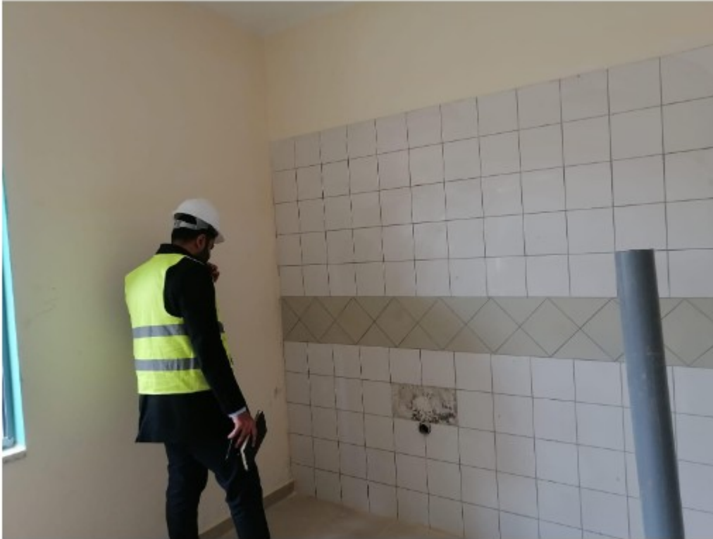
Eng. Muhammad expressed satisfaction towards wall tiling works
