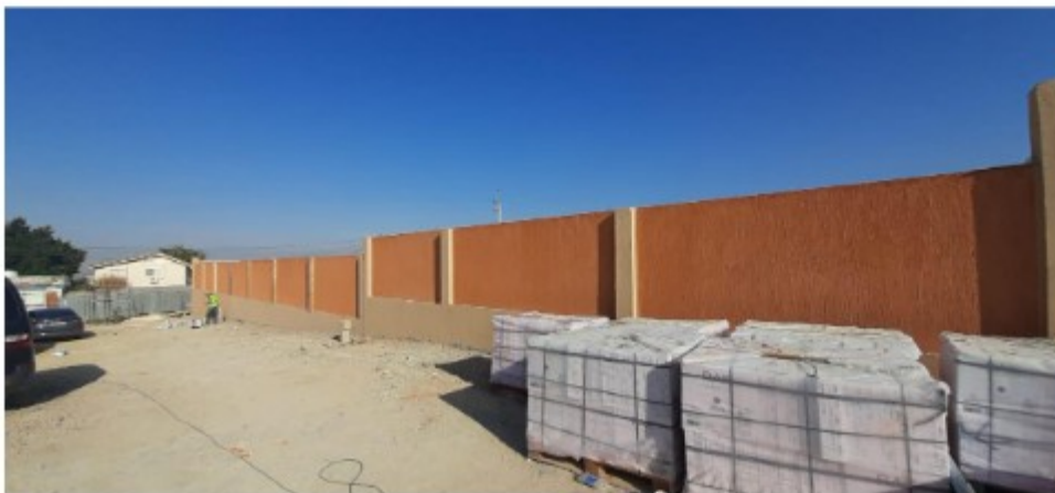
Applying colored plaster at the boundary wall
