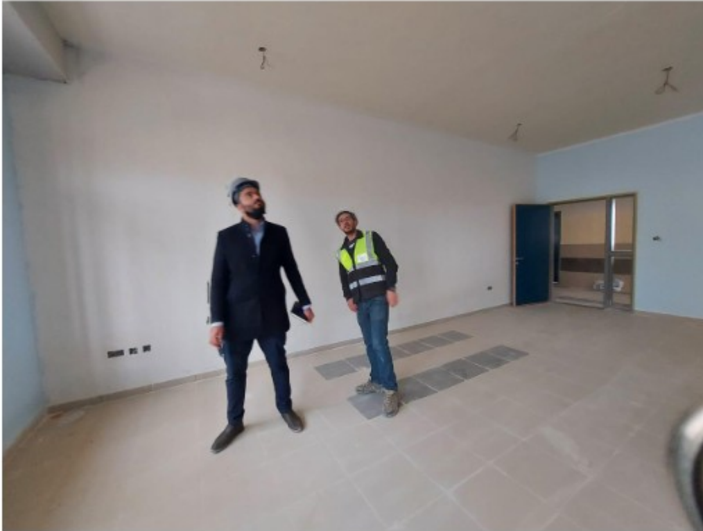
Inspecting painting work and works done on the false ceiling
