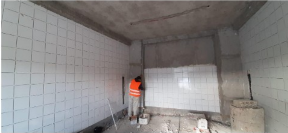
Wall tiling work at the mechanical room located at the roof
