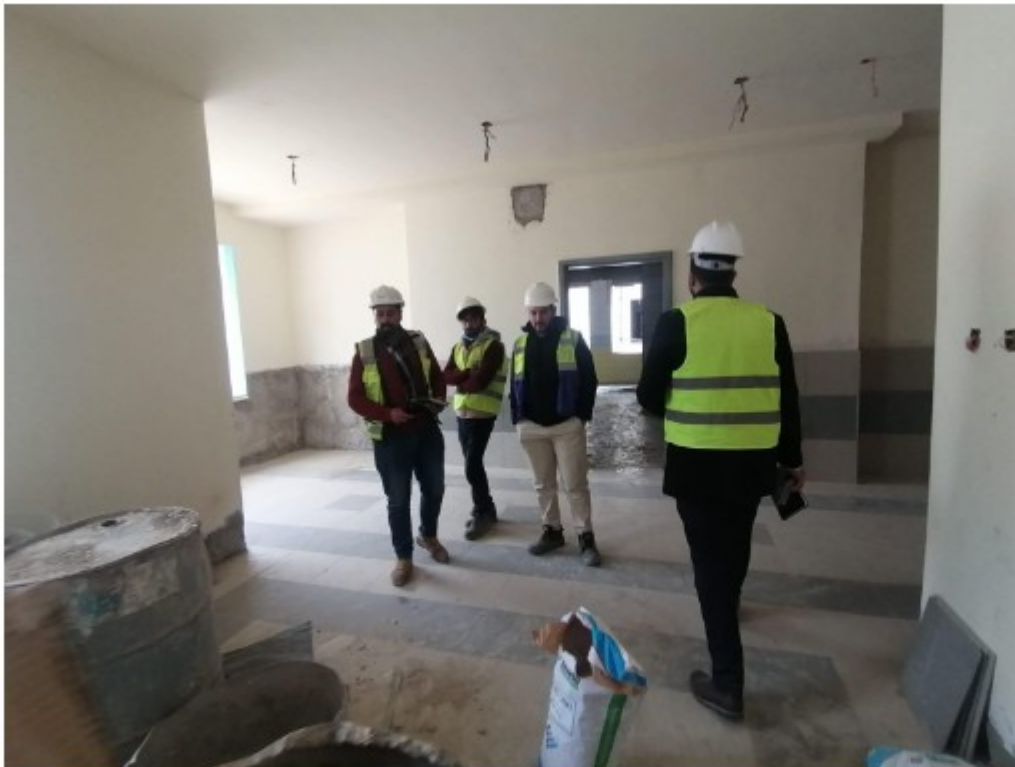
Eng. Odai recommending protecting tiles with covers used for this purpose
