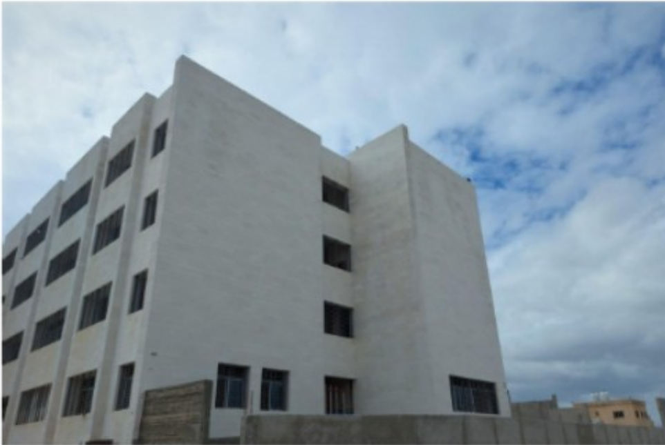
General view of the project site
