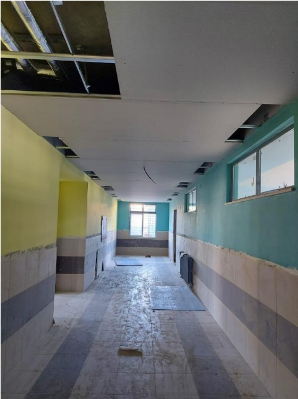
Suspended ceiling in the corridors at the ground floor
