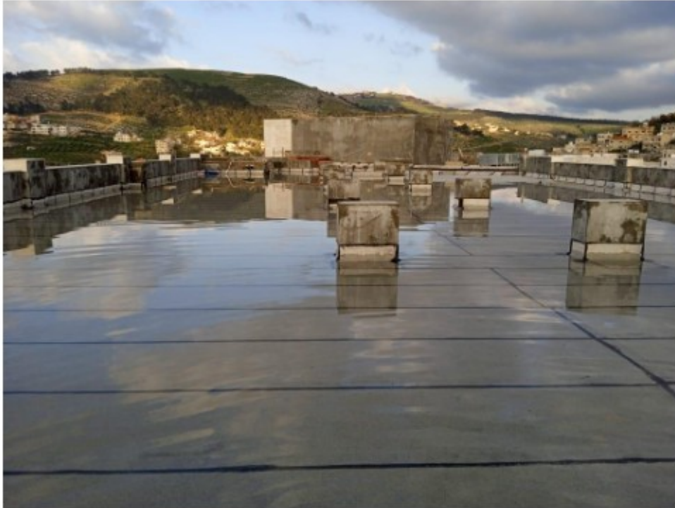
Water penetration test at the roof
