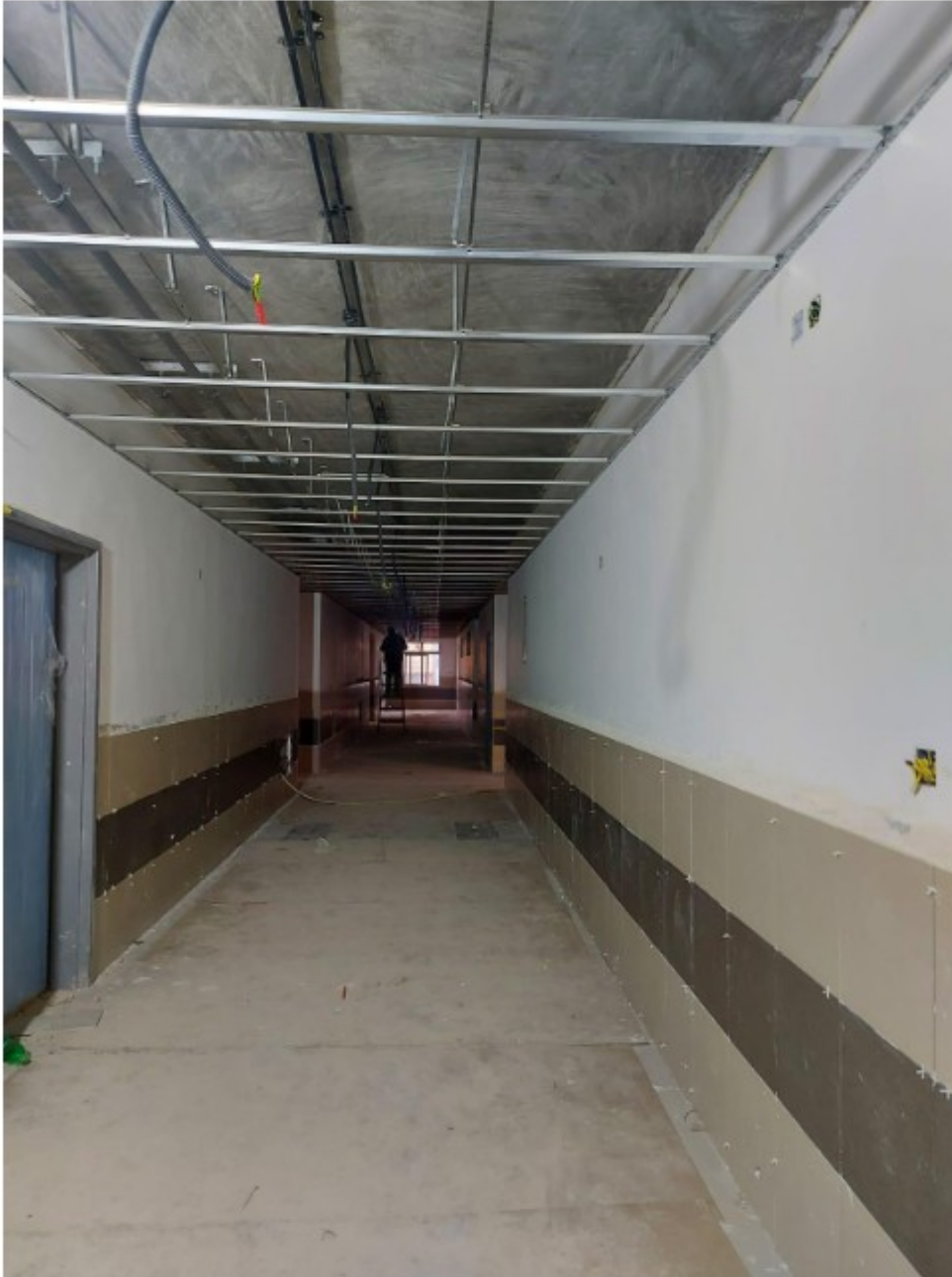
Installing the metal frame for the suspended ceiling
