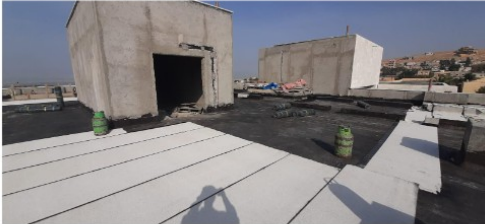
Insulation work (Waterproofing Membrane)
