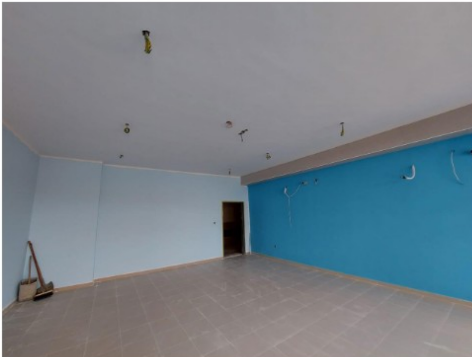
Painting and suspended ceiling at classrooms
