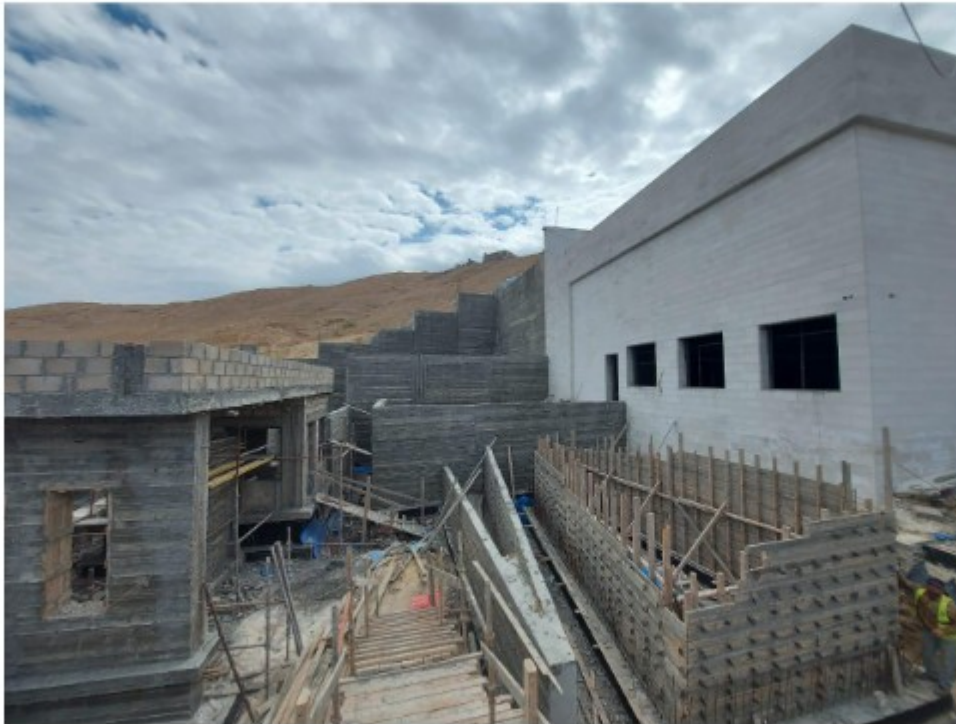
External works (guard house and ramps walls)
