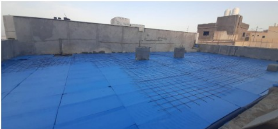
Installing extruded polystyrene and steel mesh at Zone C
