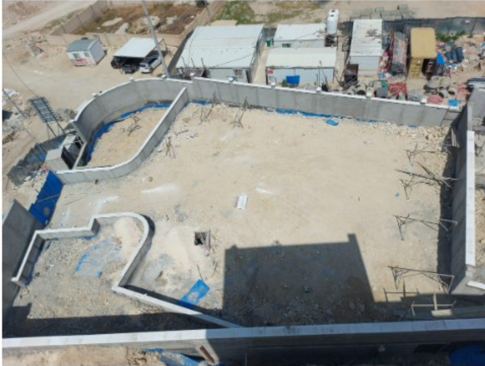
General view of a part of the external works
