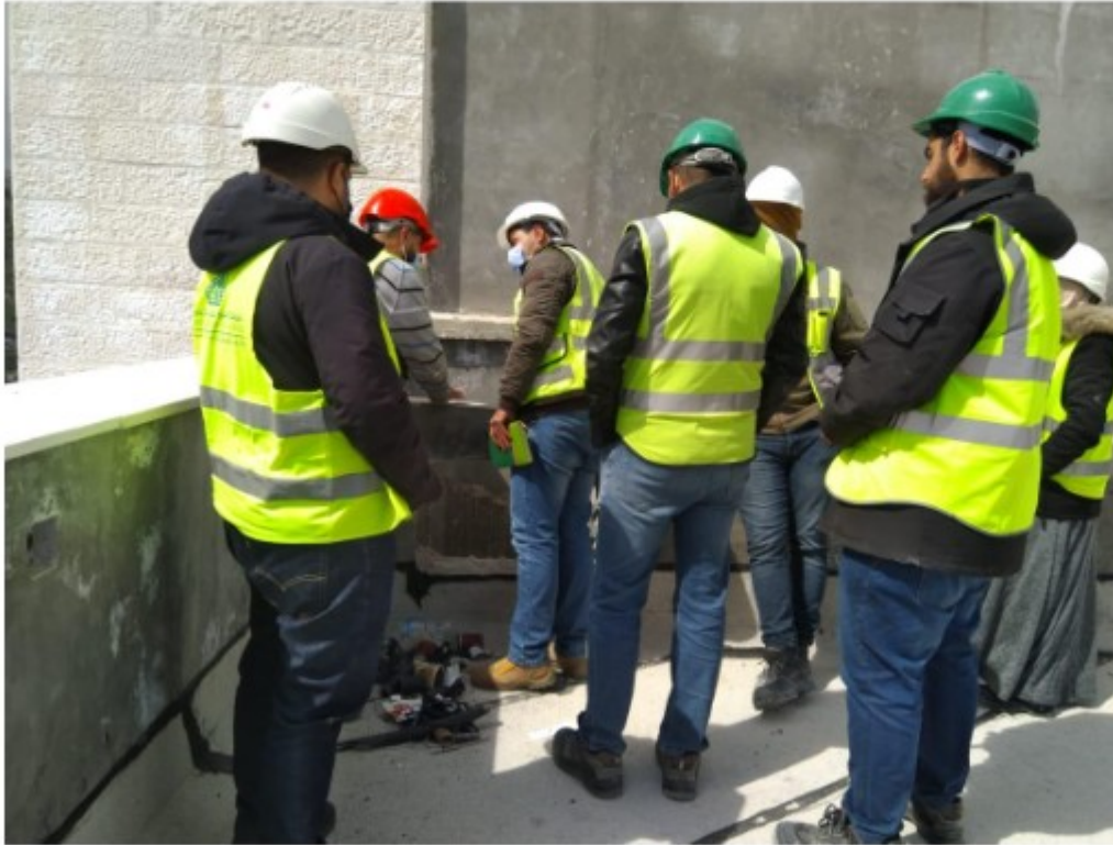
Eng. Odai recommending closing the open shaft and to use scaffoldings that abide to the safety requirements
