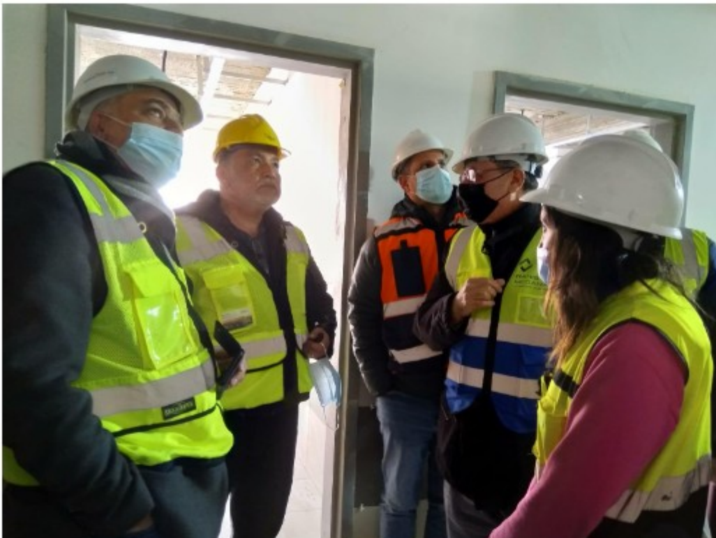
Inspecting quality at status of work.
