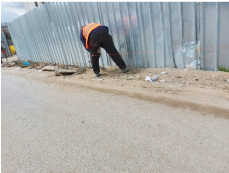
Re-installing the temporary fence according to the new plot boundary
