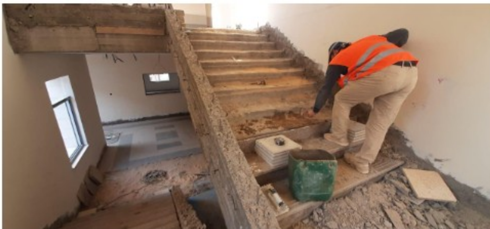
Granite tiling work at the staircase
