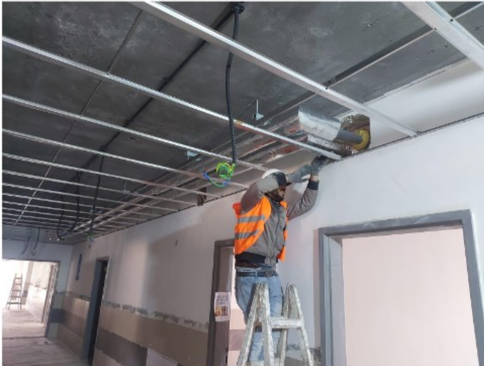
Insulation work for the heating pipes
