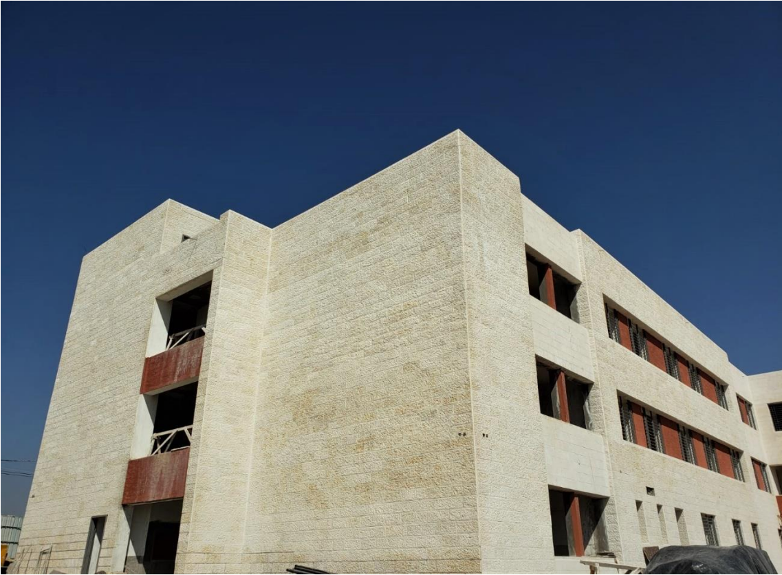
General view of the project site (Figure: 01, 02, 03 & 04)
